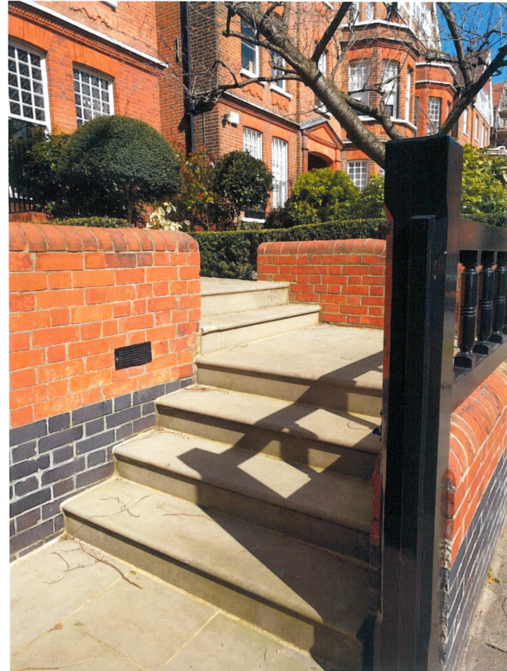
Example of Steps at 10 Wedderburn Road
