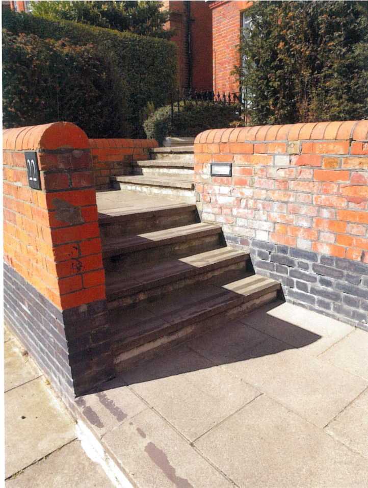
Existing Steps at 22 Wedderburn Road
