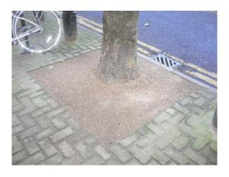
4. Detail view of London Plane (T4) with block paving displaying radial disturbance to south typically characteristic of surface root action.
