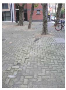
5. Detail view of London Plane (T6) with block paving displaying radial disturbance to west typically characteristic of surface root action..
