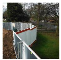
High Risk - Tree Protection Fencing (TPF1) This is to be provided by Braced Heras Fencing or solid panels. Post-holes shall be excavated by powered hand auger or low ground-pressure plant working of ground protection or outside the Precautionary Zone. Alternative more traditional post supports such as the Heras Steadfast system with an additional brace can be used where this can be pinned into position and fitted with an Anti-Tamper Coupler.
