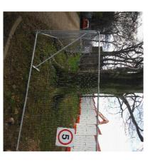
This is to be provided by Braced Harras Fencing or solid panels. Post-holes shall be excavated by powered hand auger or low ground-pressure plant working of ground protection or outside the Precautionary Zone. Alternative more traditional post supports such as the Heras Steadfast system with an additional brace can be used where this can be pinned into position and fitted with an **Anti-Tamper Coupler**.
