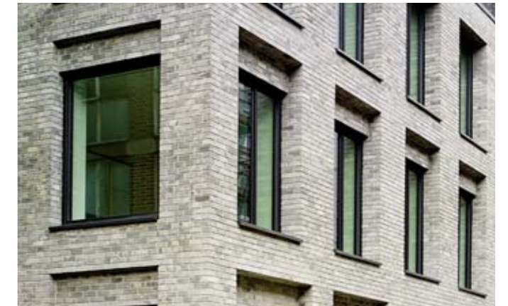
Articulated Brickwork (Charlotte Street, LBC) - DSDHA
