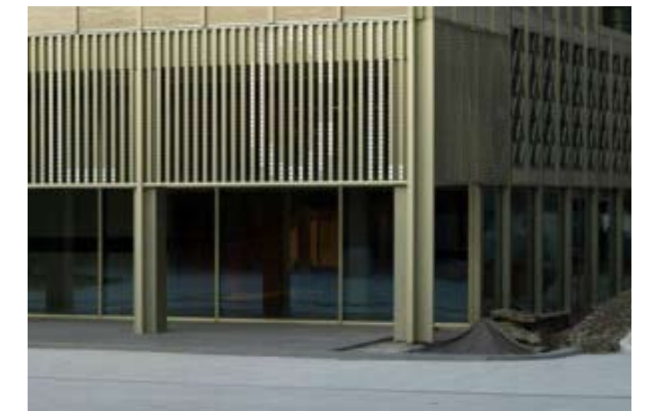
Brass-coloured metalwork at ground and first floor level
