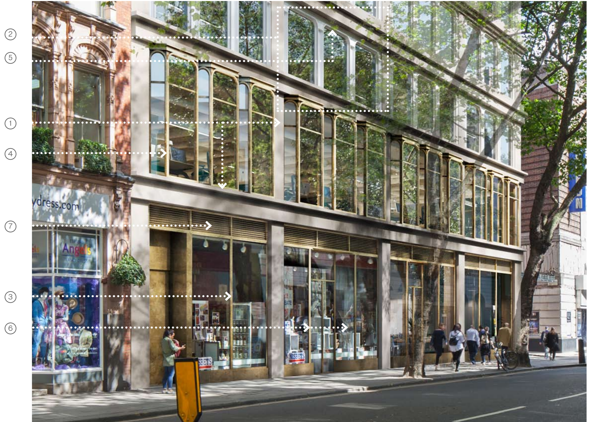
Proposed view towards new shop fronts on Shaftesbury Avenue
