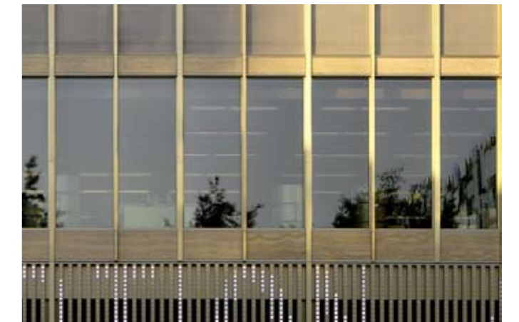
Brass-coloured metalwork at ground and first floor level
