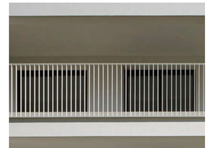
White metal work above first floor
