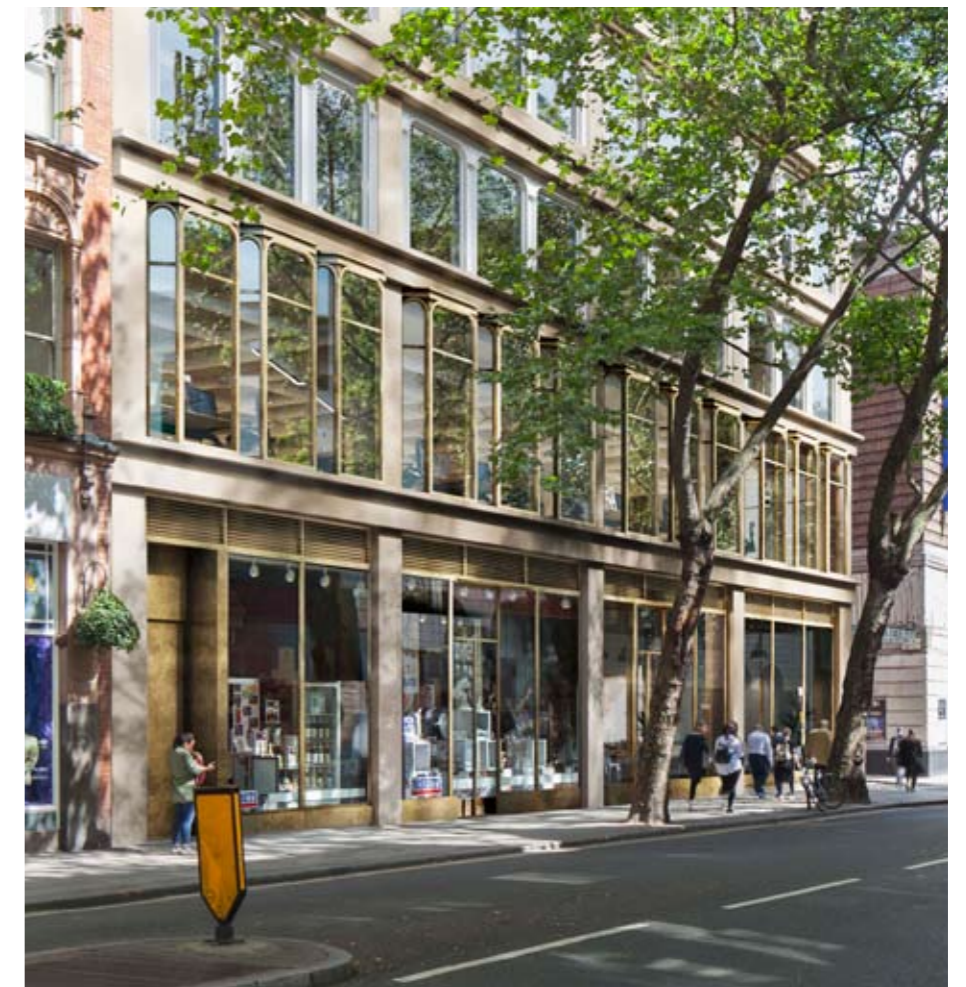
Projecting bays are used to bring delight to the first floor of Shaftesbury Avenue
