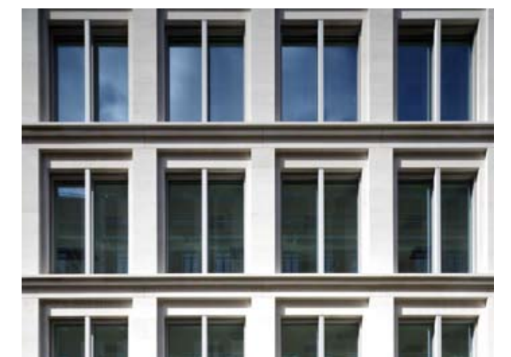
White metal work above first floor
