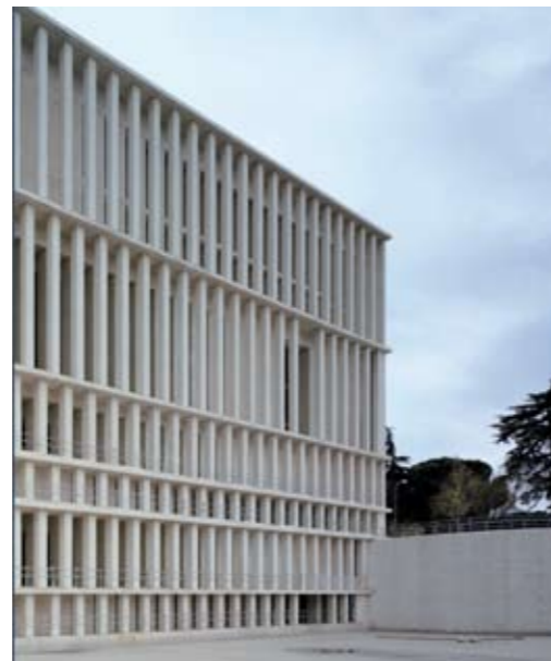
Precast Concrete Royal Collections Museum, Madrid - Mansilla+Tuñón
