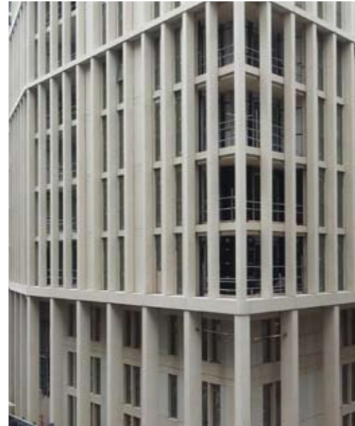
Precast Concrete Abell House, Westminster - DSDHA
