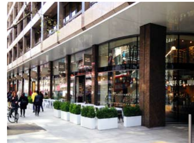
Stephen Street, ORMS (refurbishment)
