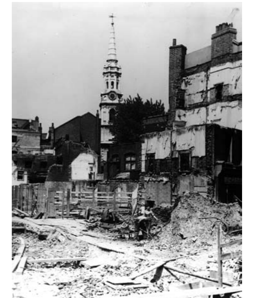
Further clearance work of the Stacey street, c.1941
