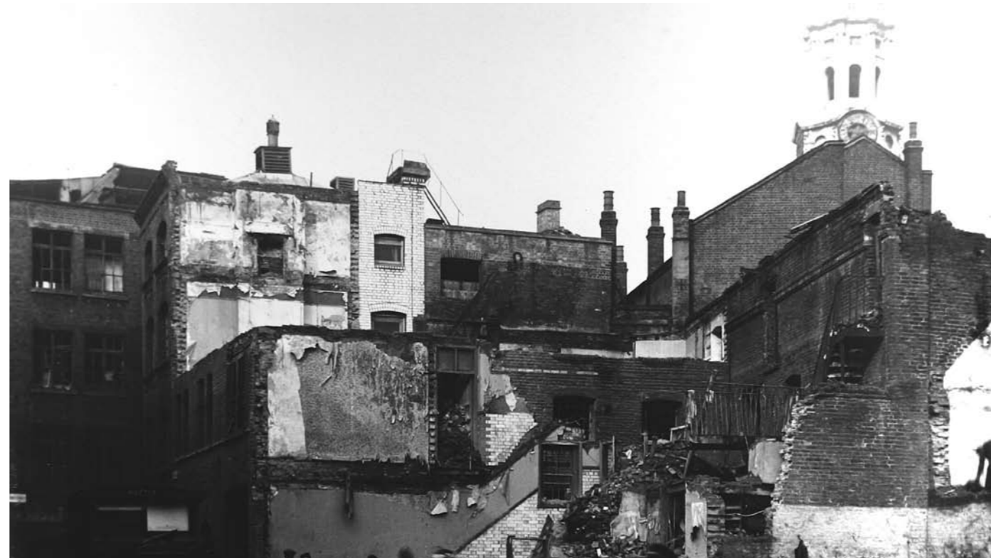
Showing the clearance of the bombed Stacey Street site
