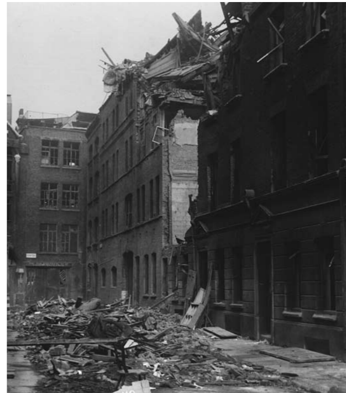
WWII bomb damage to the east side of Stacey Street
