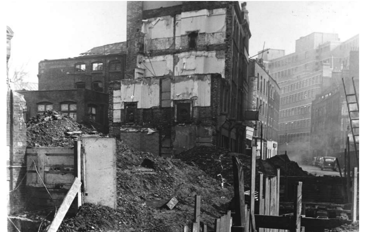
Looking west up New Compton Street, dated 3rd September 1941
