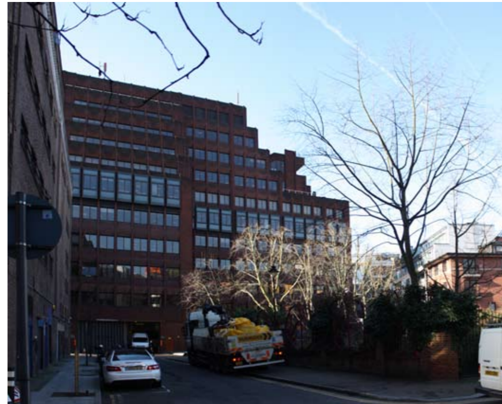
View from New Compton Street towards loading bay
