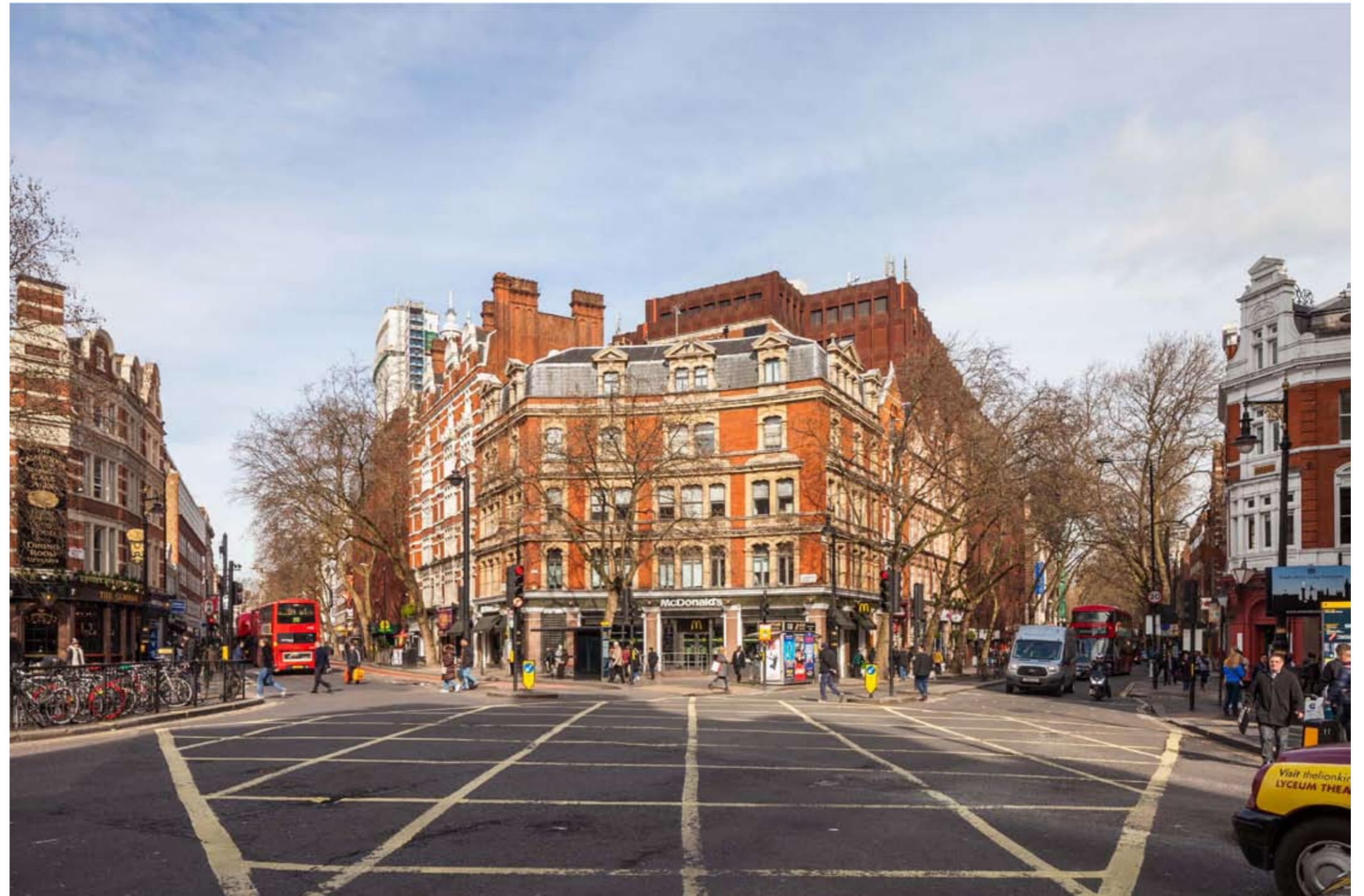
View of existing building from Cambridge Circus
