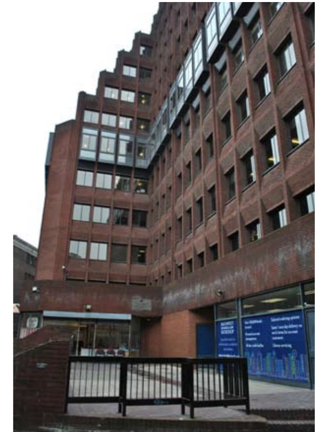
Raised public space adjacent to Phoenix Street
