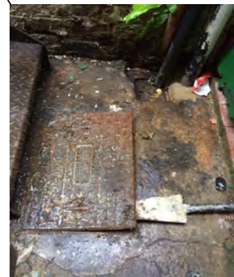
Manhole at bottom of stairs preventing trial pit.
