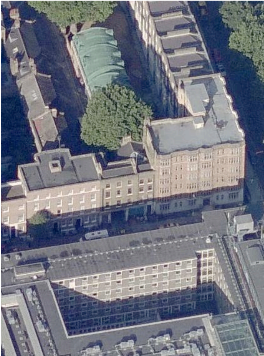
Oblique aerial view from the east
