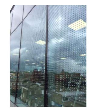
**Material Name** GL101 Clear Glazing Panel with SSAF004EX window film with externally applied white frit pattern
