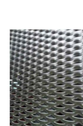
**Material Name** Expanded Aluminium Mesh set within Steel Frames
