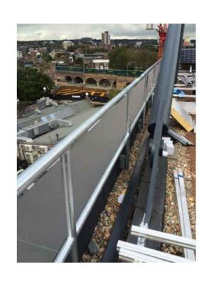
Material Name Galvanised Steel Roof Balustrade
