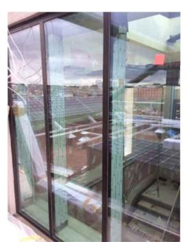
**Material Name** GL101 Clear Glazing Panel with black capping piece
