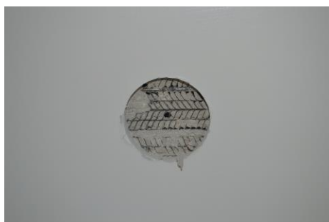
Opening up showing ceiling construction in concrete with metal laths
