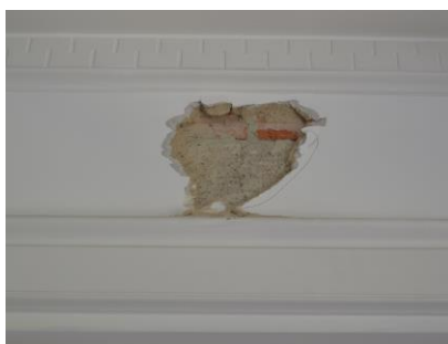
Opening up showing typical wall construction apparently in clay pot/ tile
