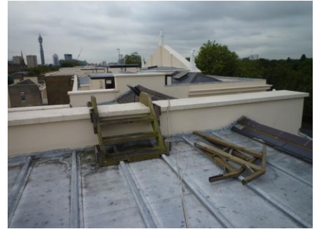
External view of rebuilt north roof with southern roof in background
