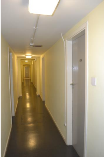
Central basement corridor
