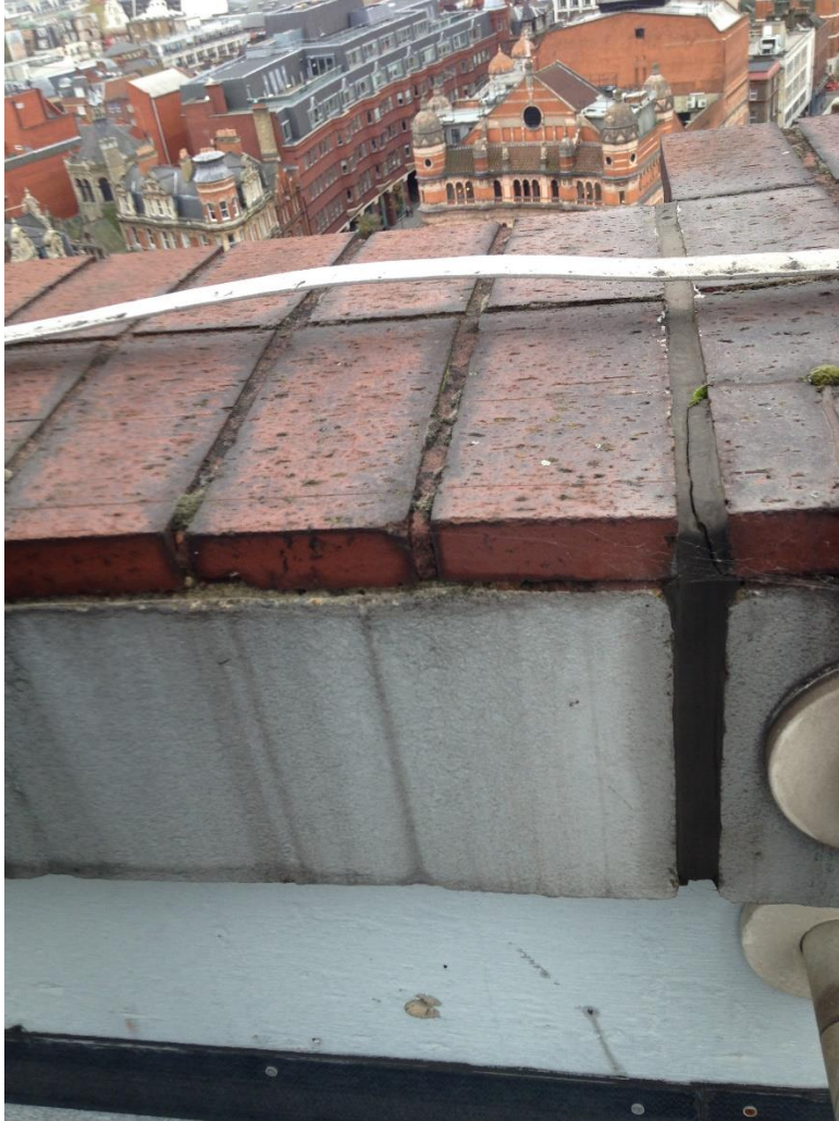
Plate 1: Single layer brick façade built over main concrete construction.
