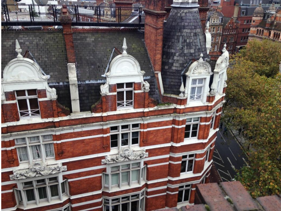
Plate 6: Adjacent Georgian building complex.
