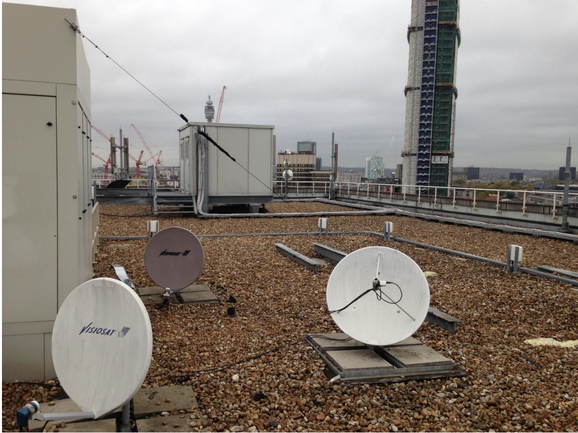
Plate 4: The top roof with gravel and concrete slab surface.
