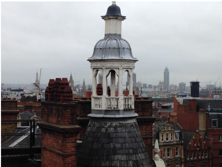
Plate 7: Turret within the Georgian building complex.
