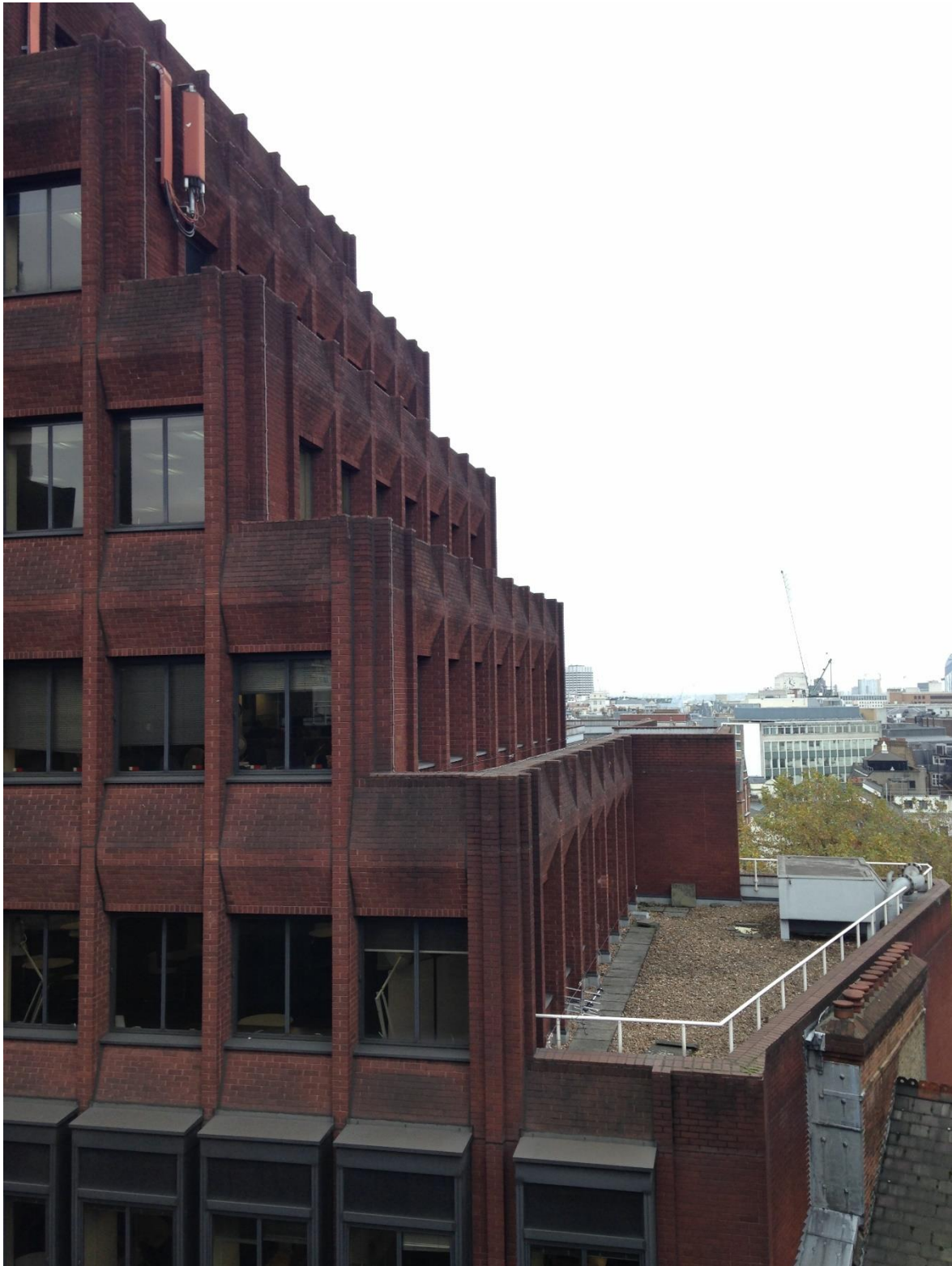
Plate 5: The south-east facing terraces with gravel and concrete slab surface.
