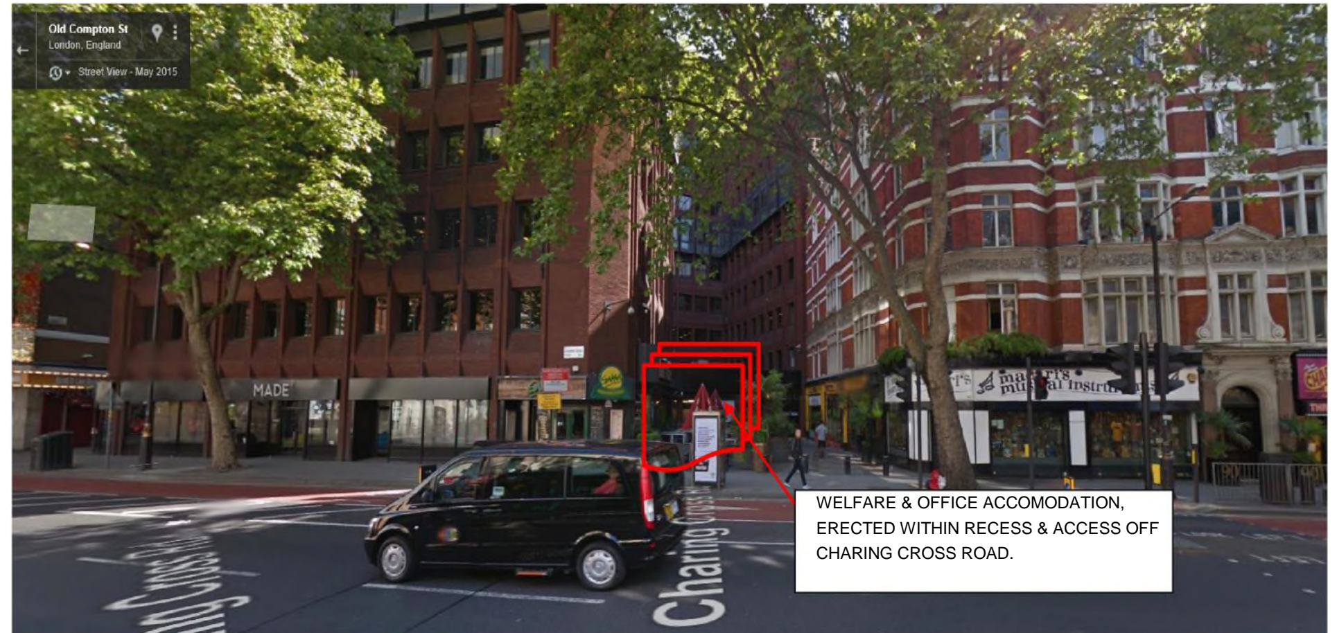
Figure 7.6 – Proposed Location of Site Accommodation during the Construction Phase of the Project
