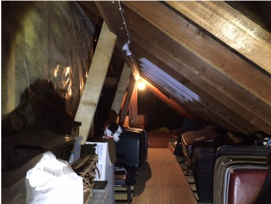
Figure 4.2 Evidence of external access into the roof void with light entering
