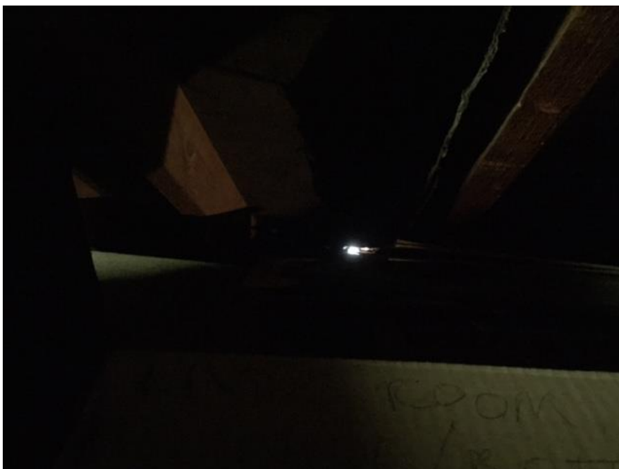
Figure 4.2 Evidence of external access into the roof void with light entering
