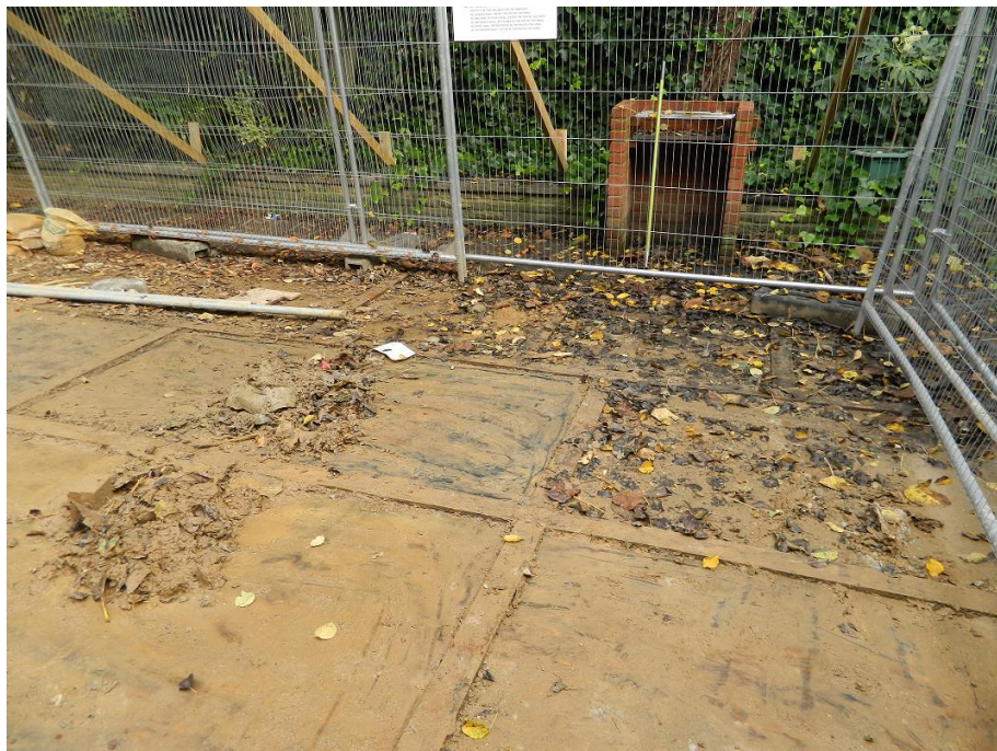
Figure 7. Plywood sheeting used as ground protection.
