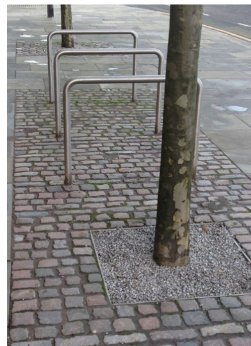
High quality granite sett detailing around Sheffield cycle stands and tree pits
