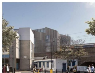
VIEW FROM WARDEN ROAD
