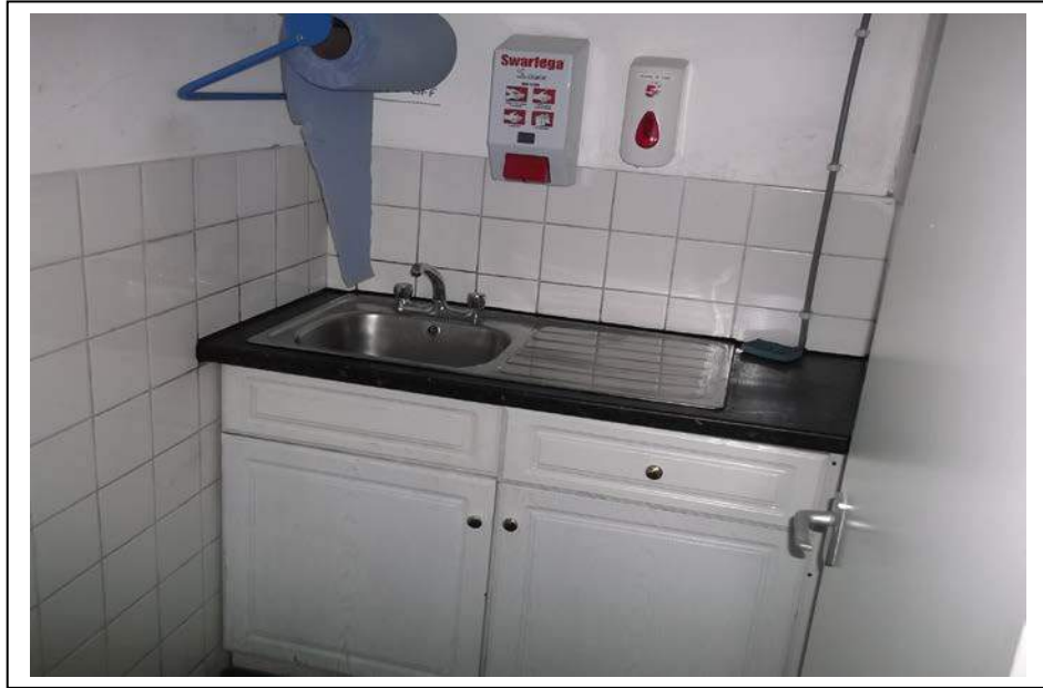
The above picture shows the kitchen with modern vinyl flooring, painted plastered and ceramic tiled walls and a plaster ceiling, a wooden door, laminate cupboards and worktop with a stainless steel sink.
