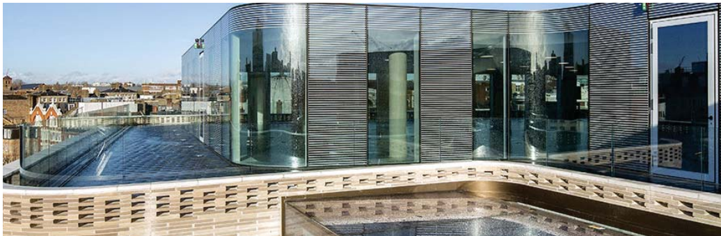
Curved curtain wall glazing system.
