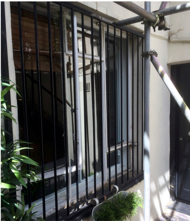
Existing Lower Ground Floor Front Window - replacement see DWG: 384(0)003
