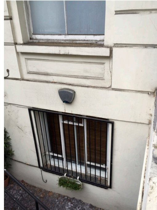
Existing Lower Ground Floor Front Window - replacement see DWG: 384(0)003
