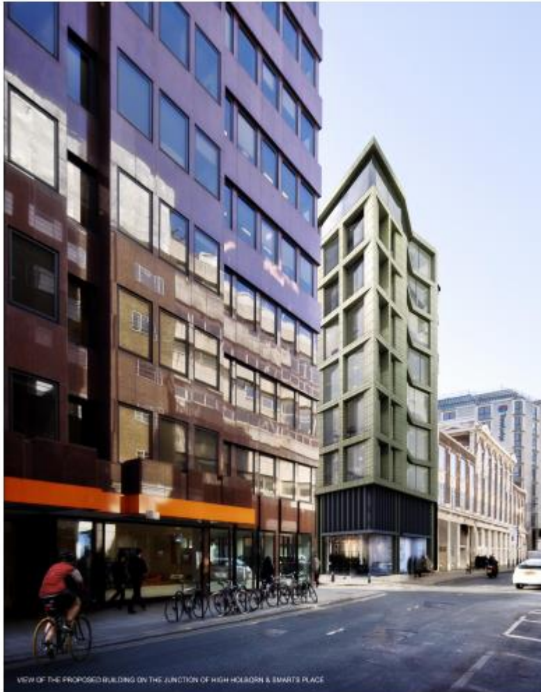
VIEW OF THE PROPOSED BUILDING ON THE JUNCTION OF HIGH HOLBORN & SMART'S PLACE
