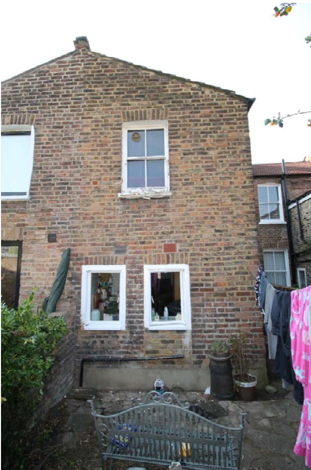
Rear of the existing closet wing
