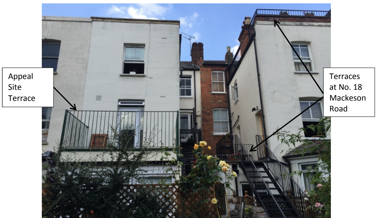
Rear Elevation of Appeal Property
