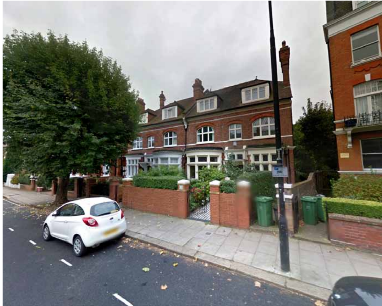
123 Broadhurst Gardens Front Elevation looking East along Broadhurst Gardens
