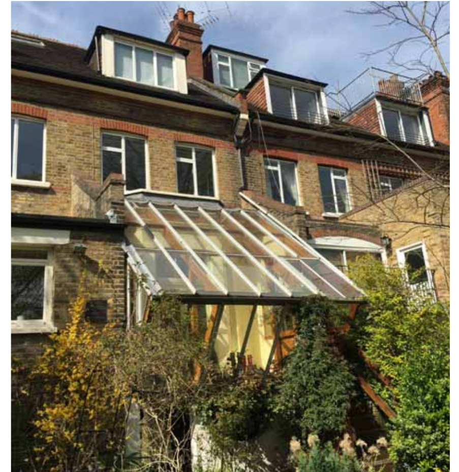
Rear Elevation Existing 'unsympathetic' glass conservatory rear extension
