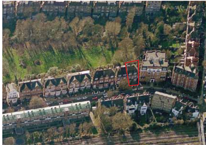
123 Broadhurst Gardens Aerial View 01 (Site outlined in red)
