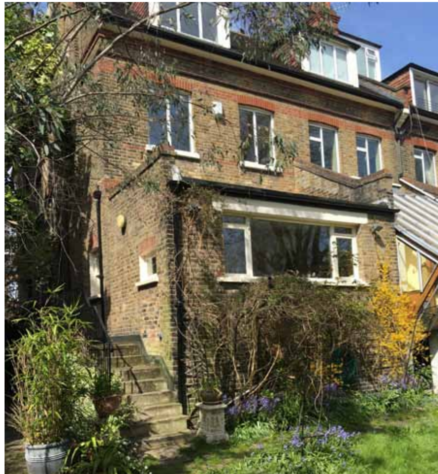
Rear Elevation Existing 'unsympathetic' rear extension
