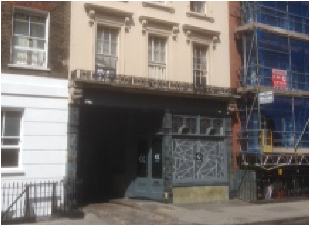
1. Front elevation – existing shopfront (37 Tavistock Place)
