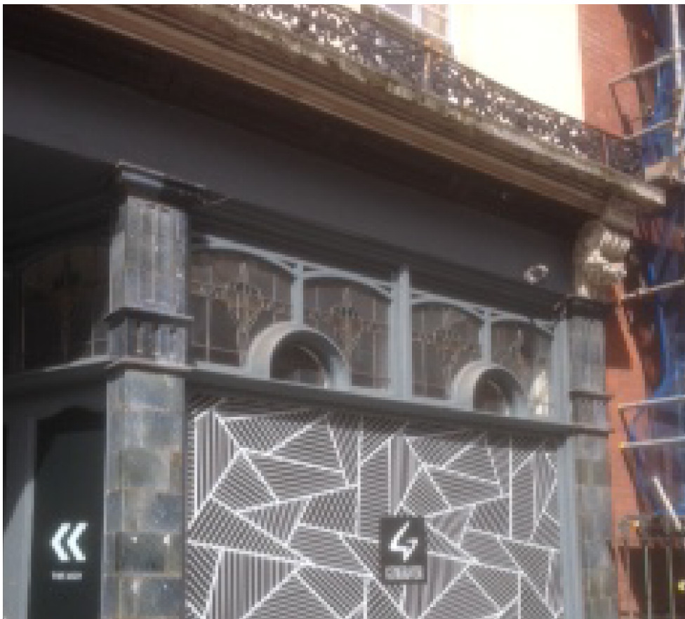
2. Front (right) – hanging sign will be fixed below right-hand cornice / illuminated lettering on fascia board beneath overhanging balcony
