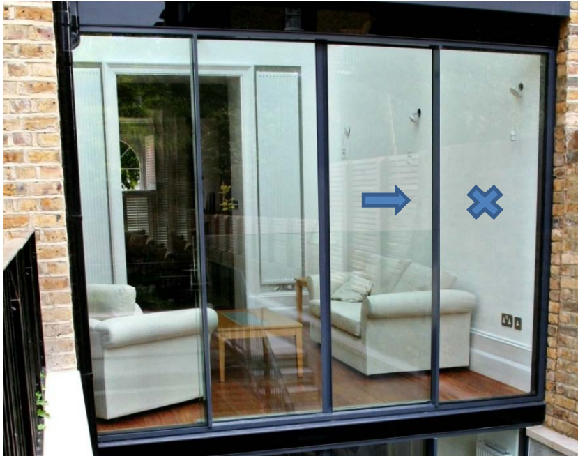
Pic. 5: Example of window type B
