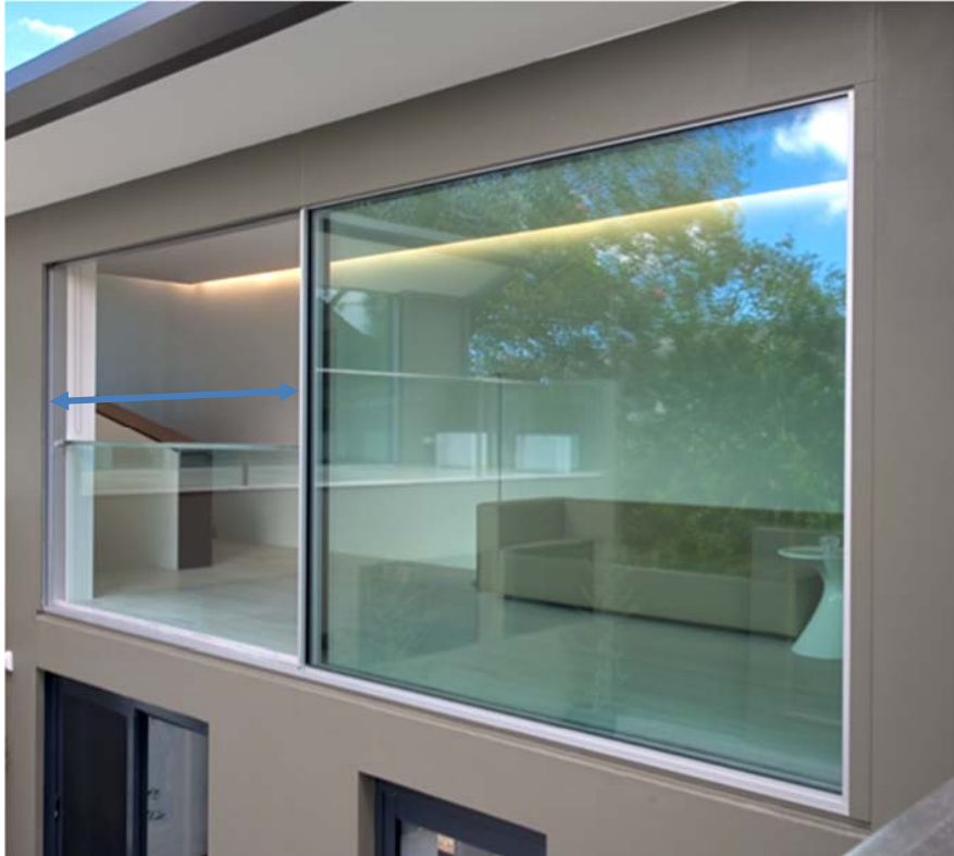
Pic. 2: Example of railing type 02
