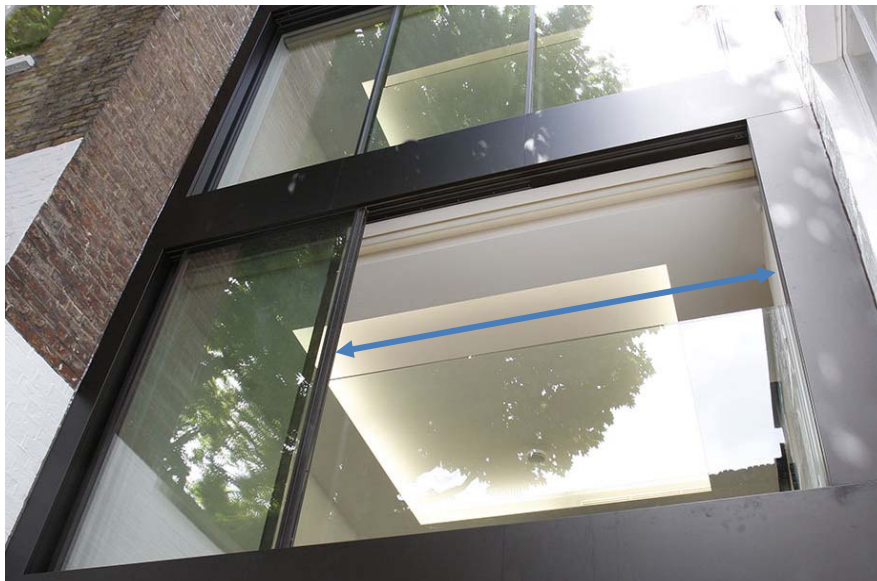
Pic. 1: Example of railing type 01
