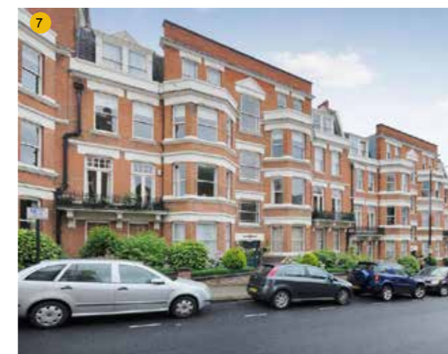
7 Period Mansion blocks that line West End Lane further North.
