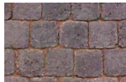
ST2: Permeable Paving
