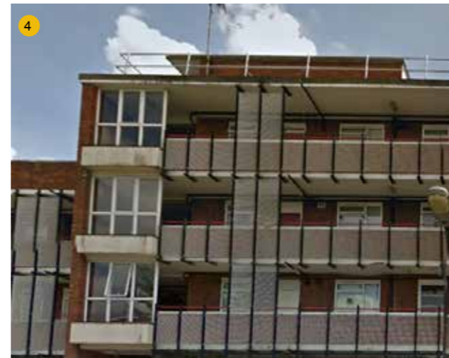
4 Vertical banding - 1960s Holmesdale House
