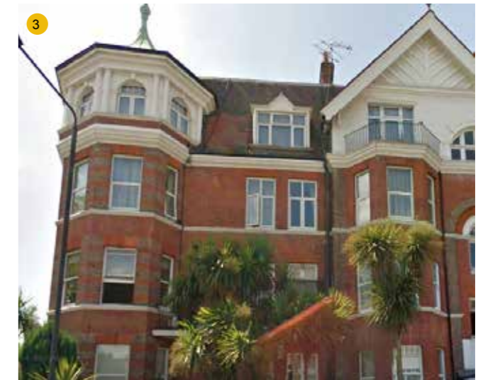
3 A neighbouring mansion block showing generous fenestration and grey slate roofing.
