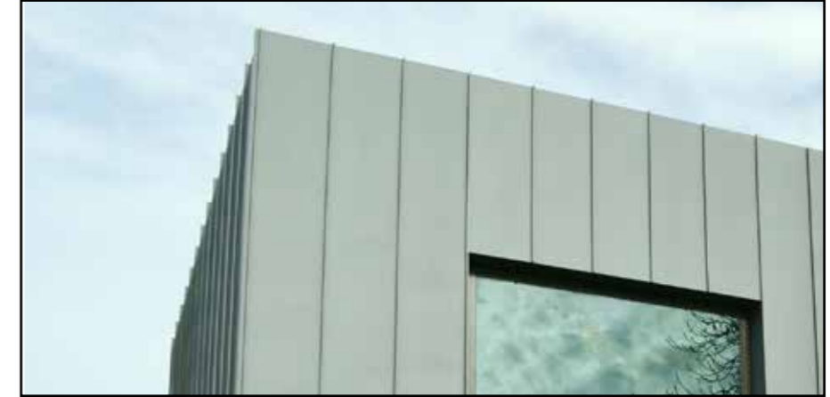
Seamless standing seam zinc facade with deep window reveals
