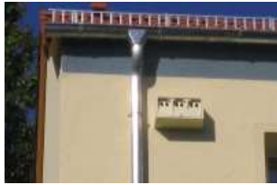
[Pic. 6]: Example of installed 1SP
