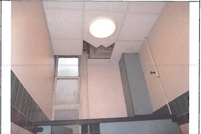
Photo 4: Existing Room 125B suspended ceiling, metal window, tiled and decorated walls.
