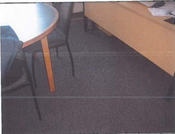
Photo 19: Existing room 221 roll carpet floor.
