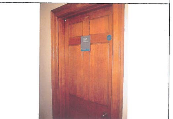
Photo 16: Existing room 221 solid timber door, to remain.
