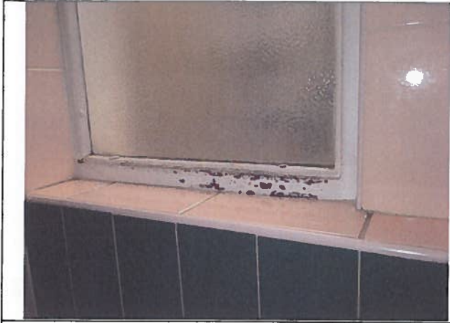
Photo 11: Existing internal tiled cills.
