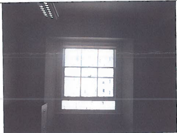
Photo 20: Existing room 221 sliding sash timber windows with single clear glazing.
