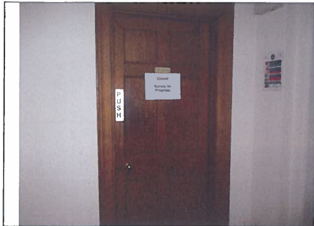
Photo 1: Existing door leading from North Cloister corridor to Room 125 – to remain
