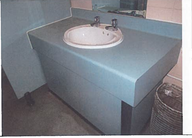
Photo 6: Existing Room 125B wash hand basin, vanity unit and vinyl floor covering.
