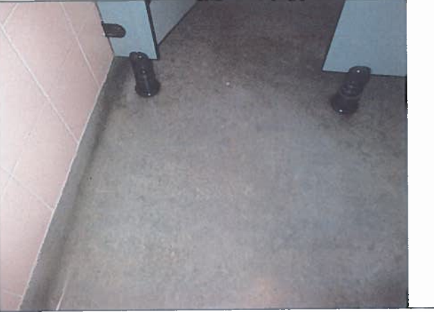
Photo 10: Existing Room 125C floor covering and tiled wall.
