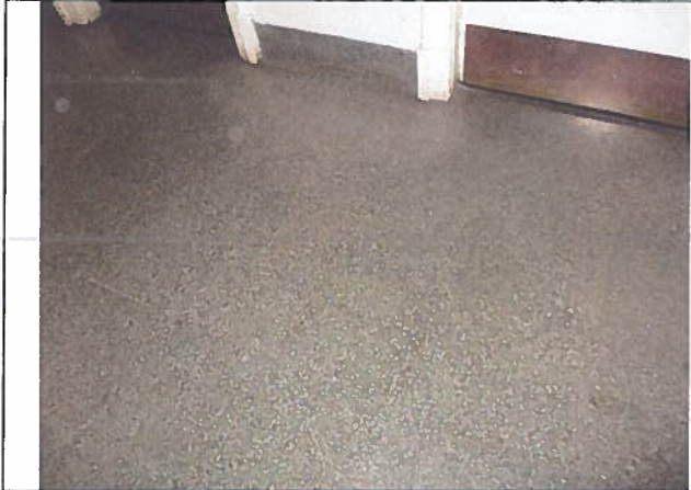
Photo 3: Existing Room 125 tiled floor covering with upstands.
