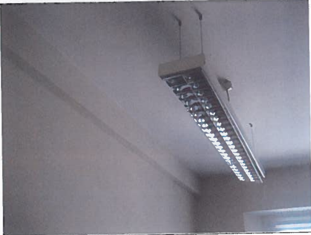
Photo 17: Existing room 221 hung strip lights and decorated plaster walls and ceiling.
