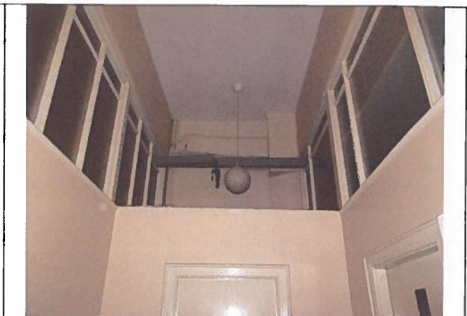
Photo 2: Existing Room 125 ceiling and high level borrowed light windows. The windows located on the North Cloister corridor are to be remain, whereas the windows opposite to be removed.
