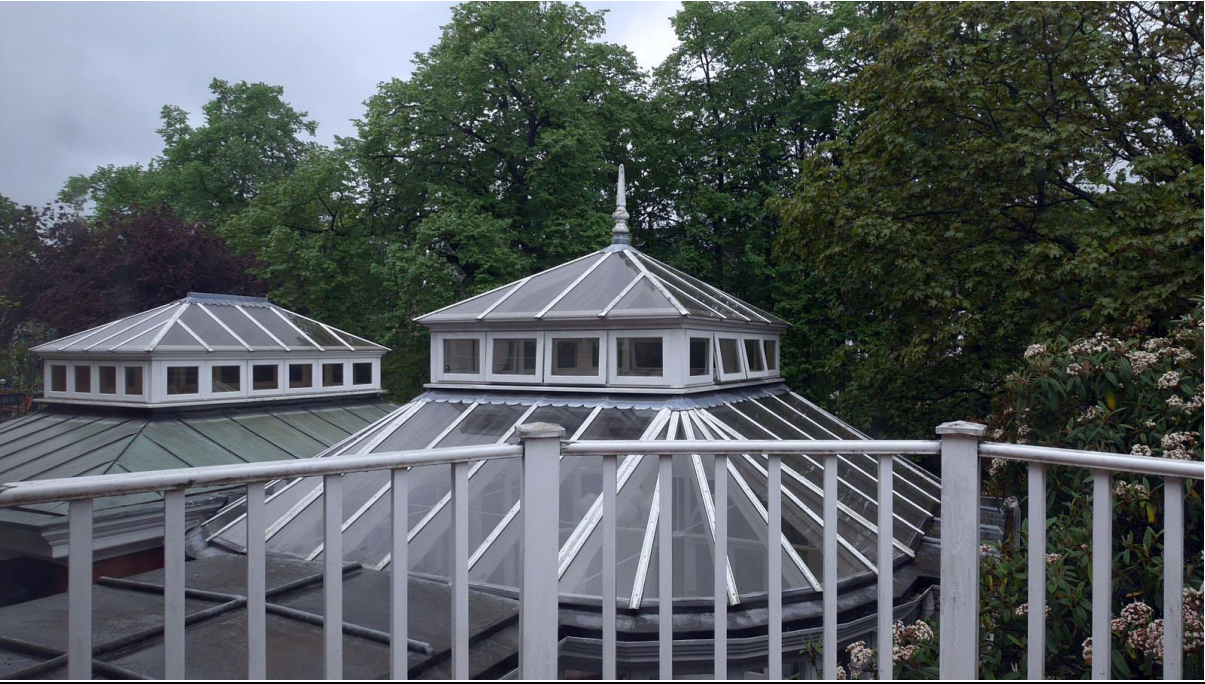
Conservatory roof (centre) at rear of house
