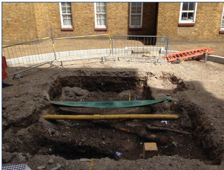
Photo 3: Service at 300mm below existing ground level of planting location 2.
