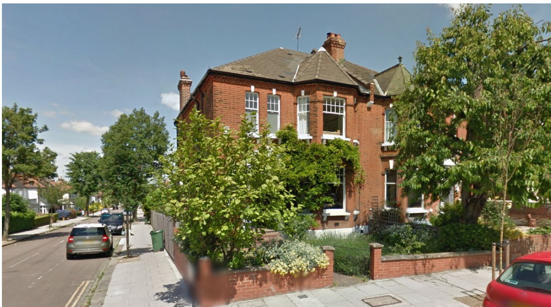
photo 1 – front facade with immediate site context; viewing from Minster Road
