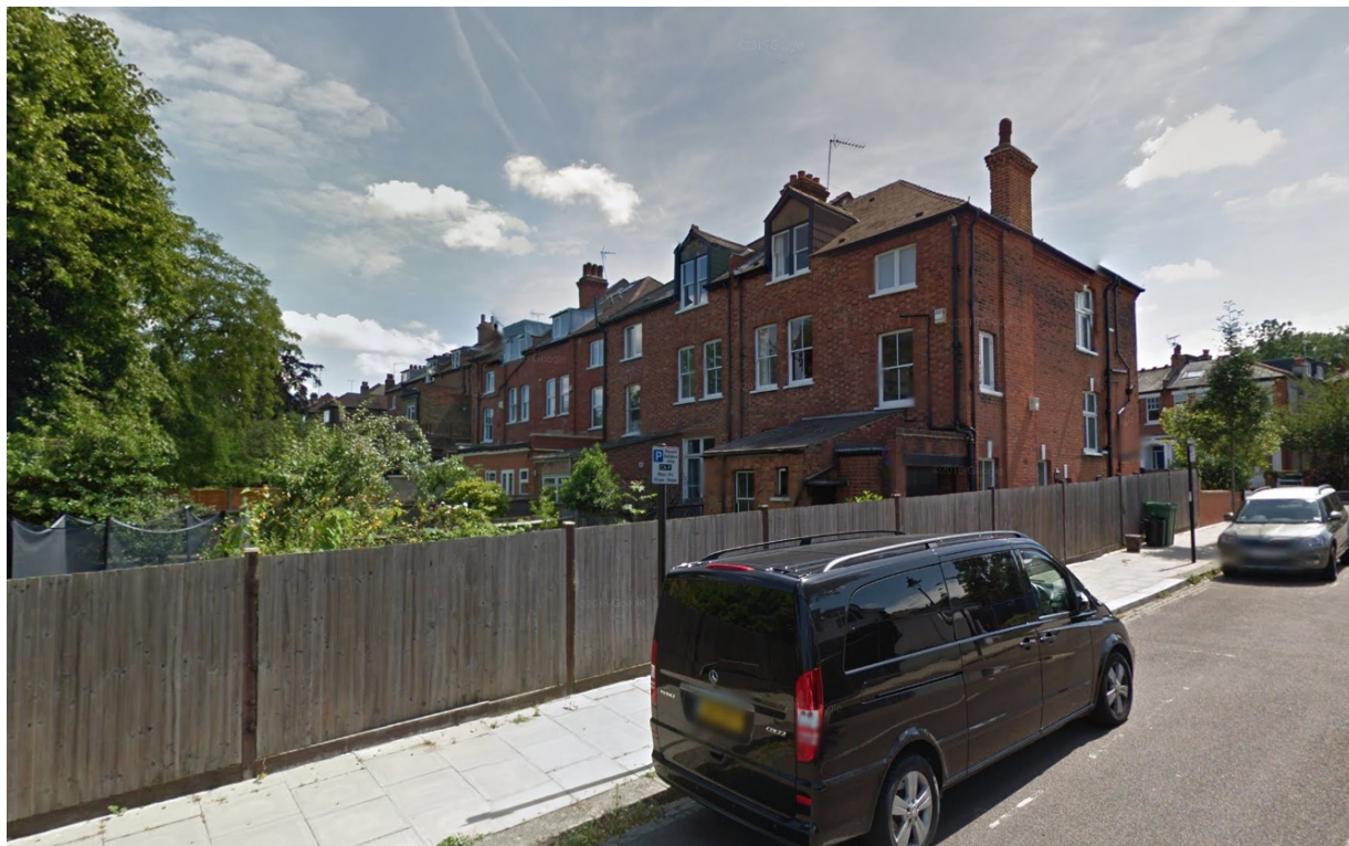
photo 2 – rear and side elevations fronting Asmara Road
