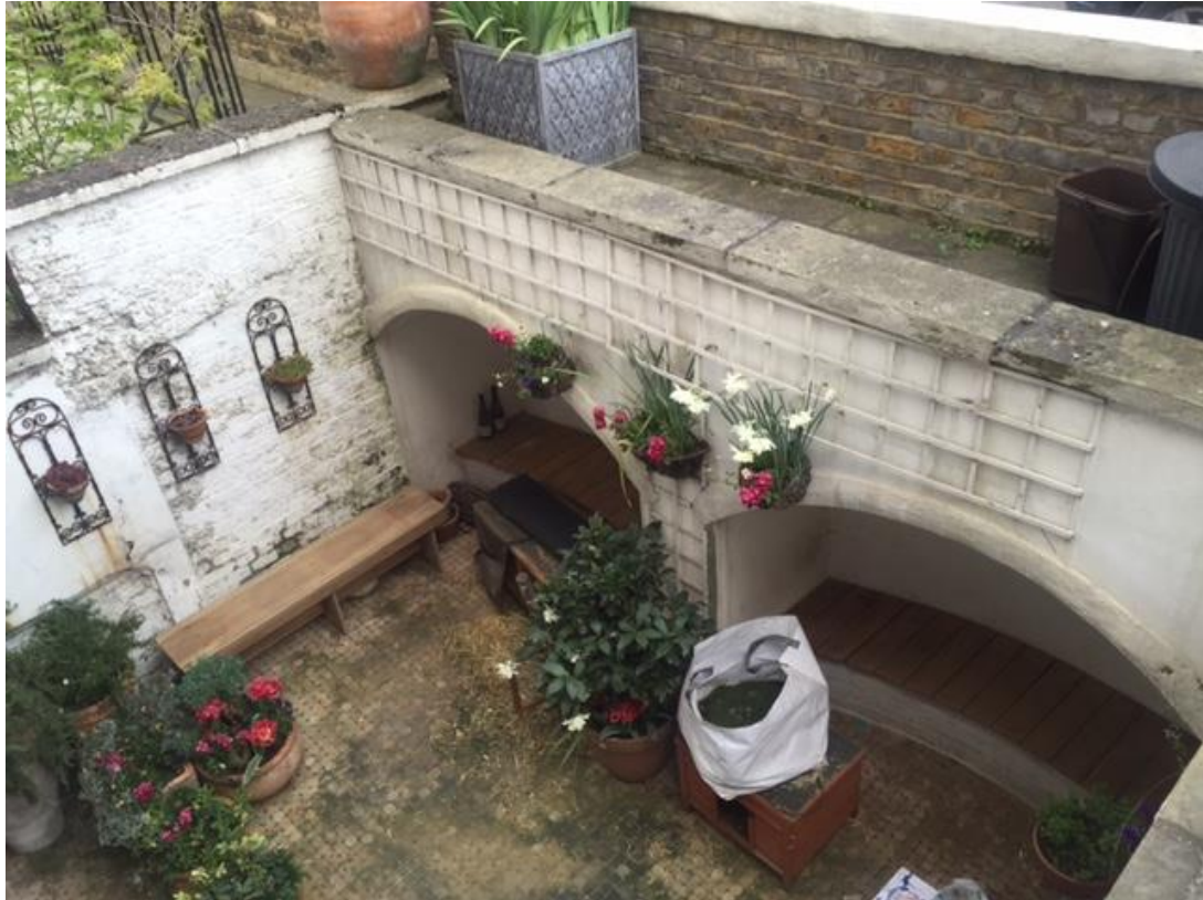
Photo 3: Front lightwell and vaults
