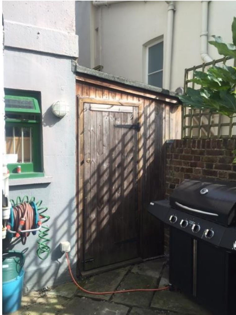
Photo 13: Existing lean-to extension
