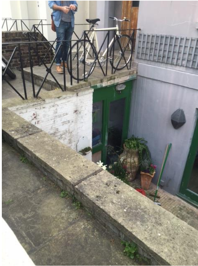
Photo 1: Front lightwell and entrance door
