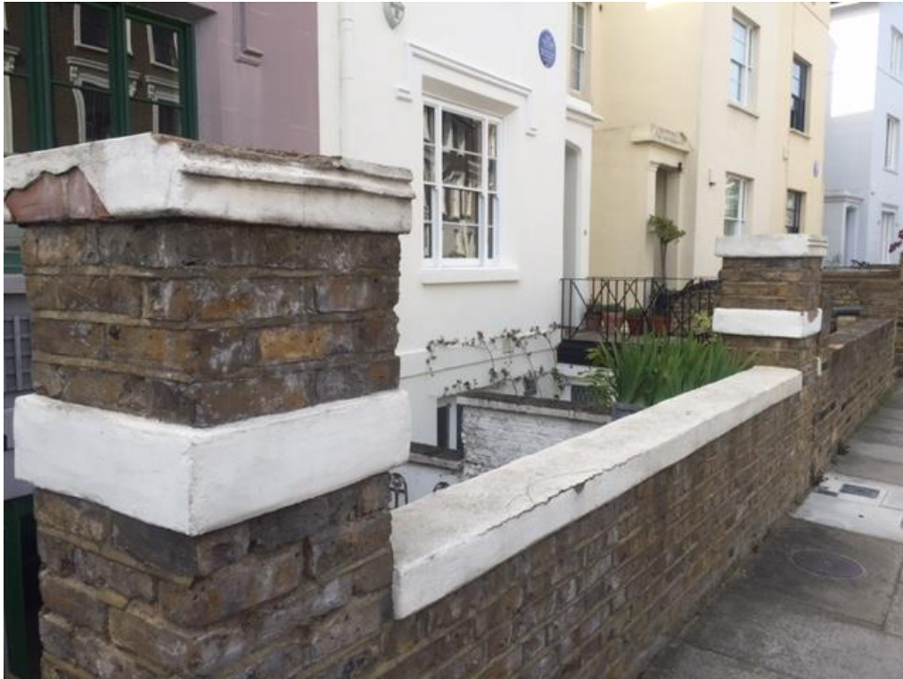
Photo 5: Existing front boundary wall at application site
