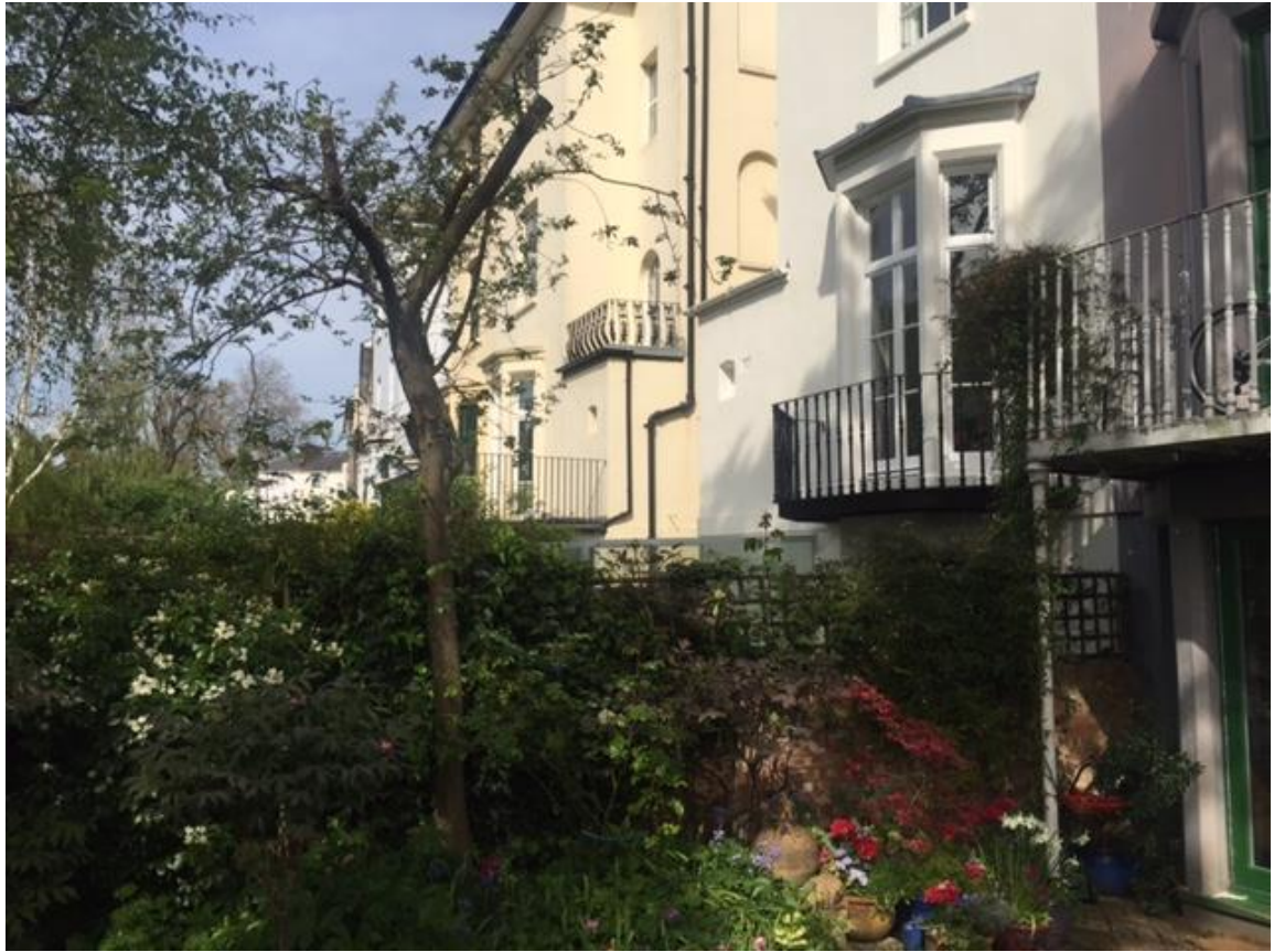
Photo 11: Rear elevation of no.13
