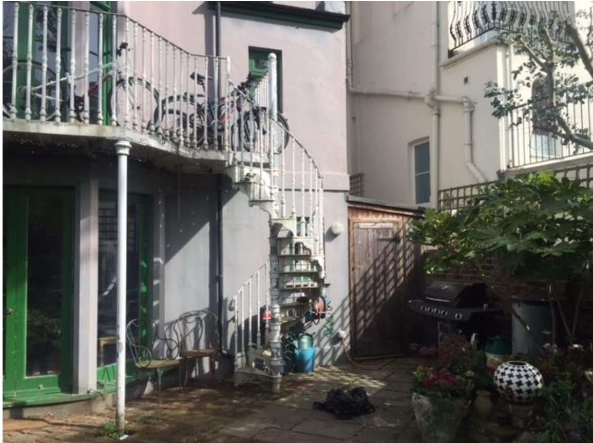
Photo 9: Rear elevation and existing lean-to extension
