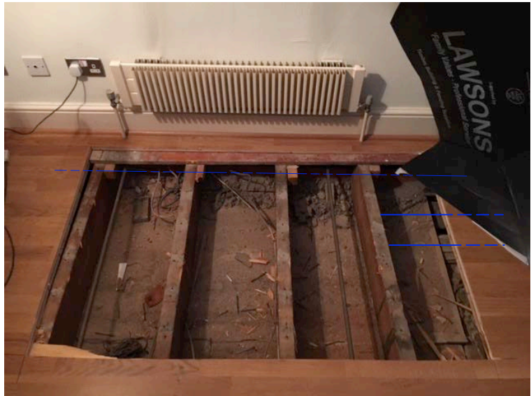
Angle edge beam to support floor joists
