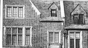
Designed to replicate traditional putty glazed steel windows, they are slim-line and just 32mm deep. They have a 45° chamfered sash design, are highly secure and have a range of authentic furniture options.
