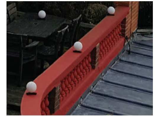
Existing Balustrade to Flat 8 Terrace 1.
