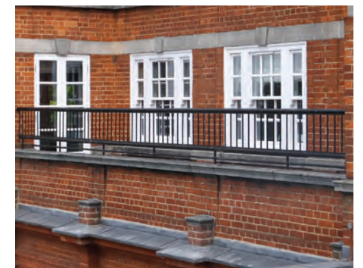
Wrought Iron Balustrade to House 2 Terrace.
