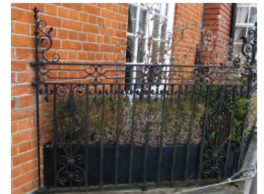
Wrought Iron Balustrade to Flat 8 Master Bedroom Terrace.
