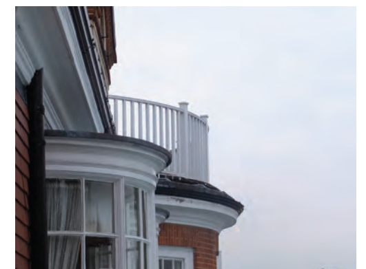
Timber Balustrade to Flat 12 Terrace.
