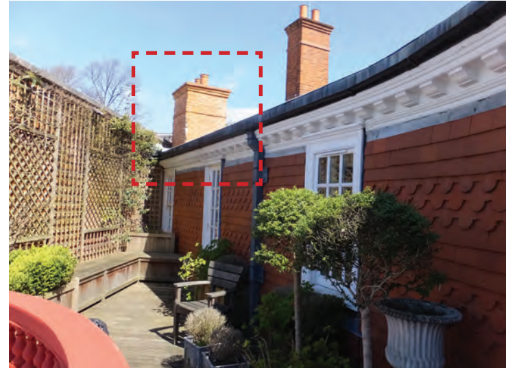
Current False Chimney. Site photos 2016. Charlton Brown Architects.
