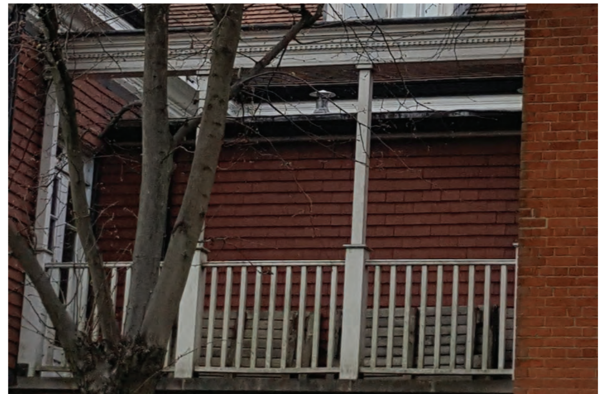
Existing Terrace - Street View.
