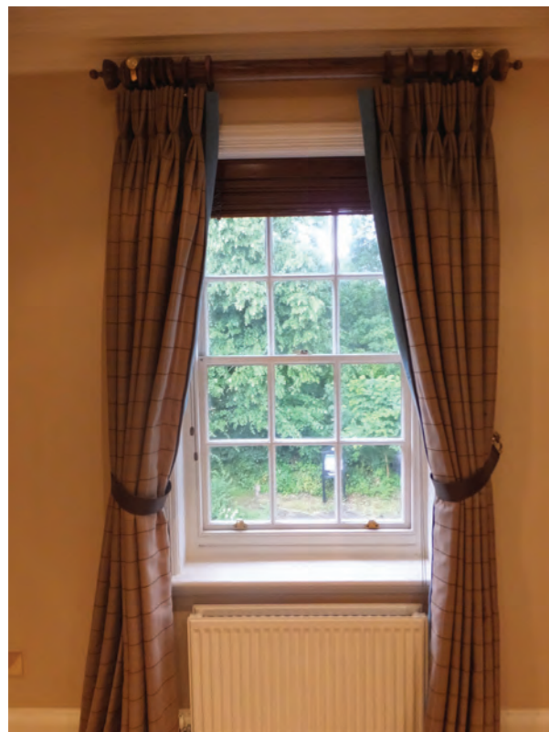
Existing Sash Windows to Study, W.C, Bedroom 2 & Ensuite.
