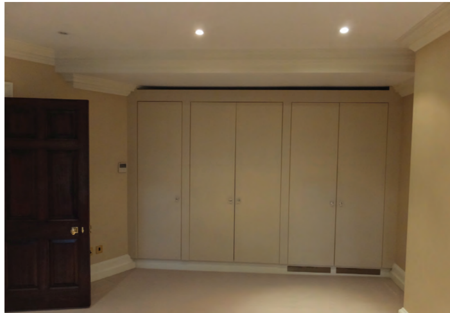
Existing Study Drop Ceiling and Built in Cupboards.
