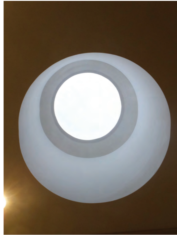
Existing Guest W.C. Skylight.
