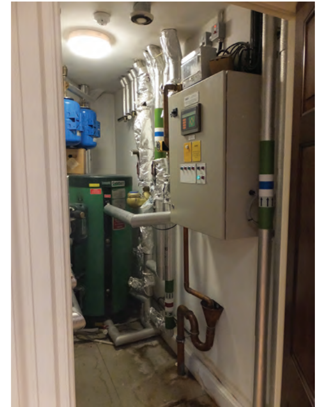
Existing Plant Room
