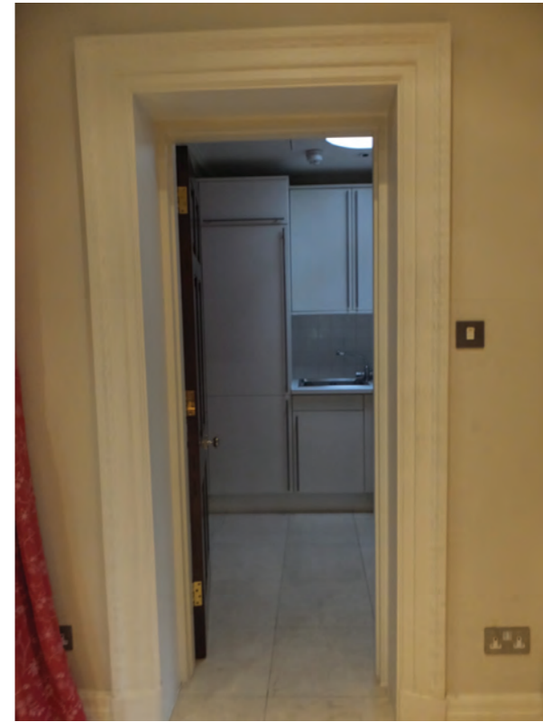
Existing Utility off Kitchen
