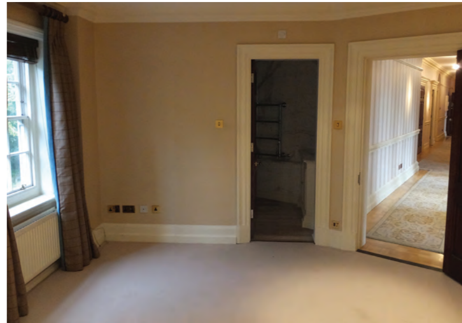
Existing Study - View back to Hallway.
