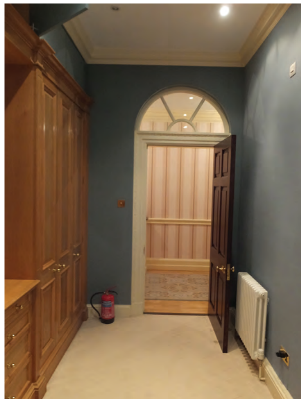
Existing Dressing Room Door Fan Light.
