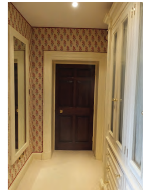
Existing Lowered Ceiling in Master Dressing.
