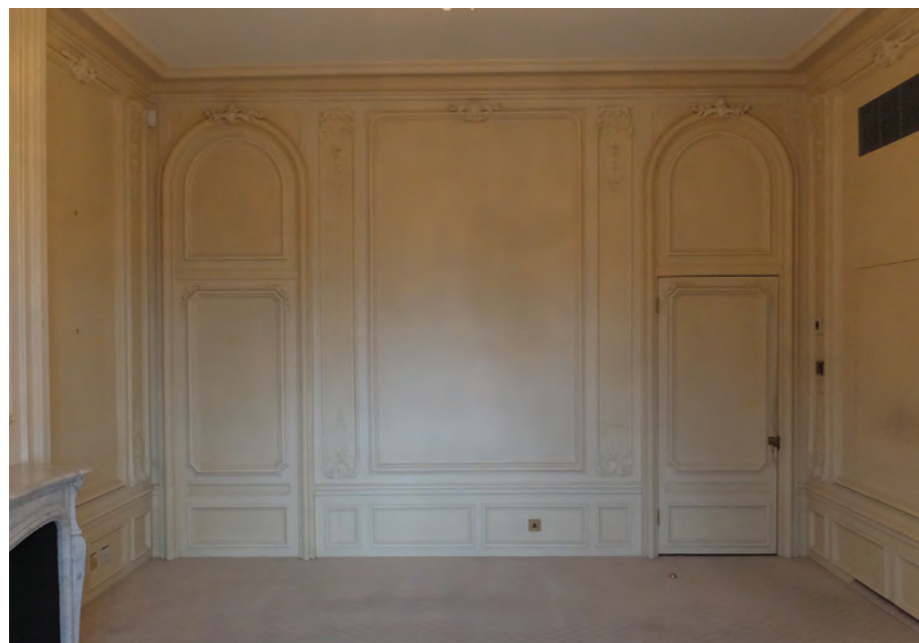
Existing Jib Door to Master Bedroom from Hallway
