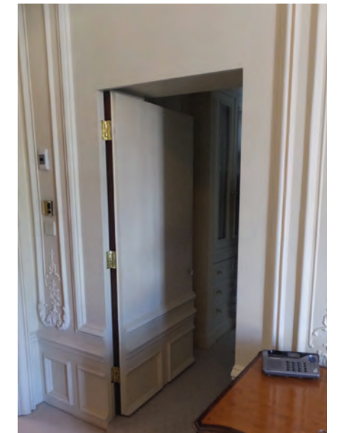
Existing Jib Door to Master Dressing.
