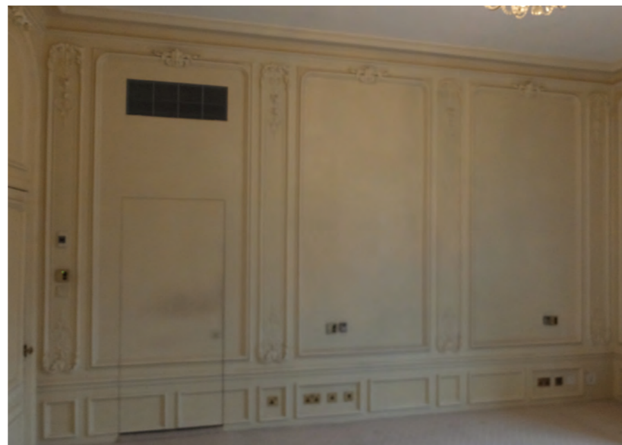
Existing Jib Doors to Master Ensuite
