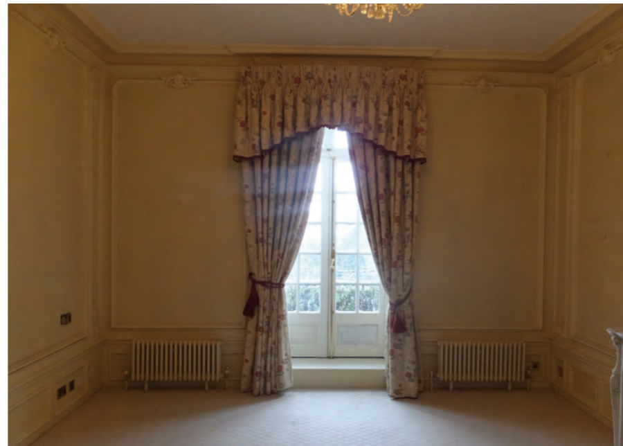
Existing Door to Terrace in Master Bedroom.
