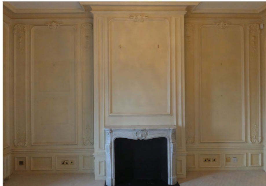
Existing Master Bedroom
