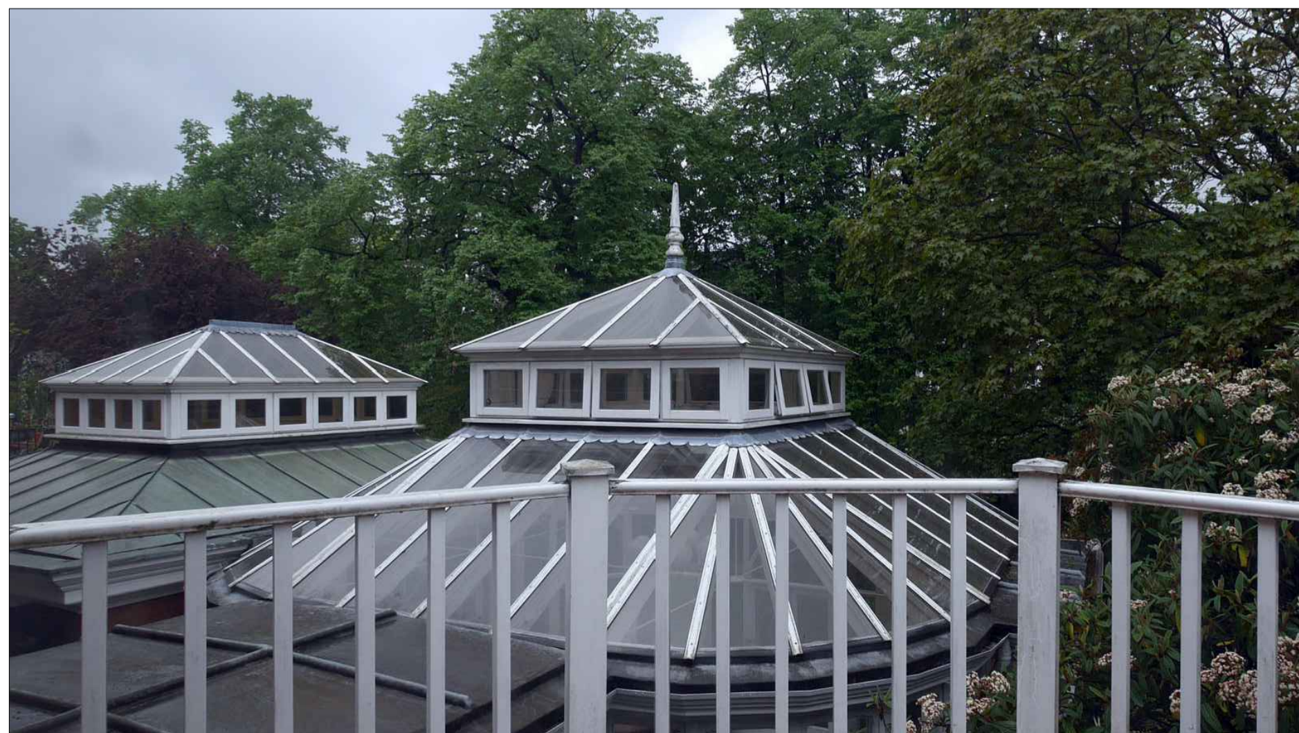
ROOFS AT REAR
