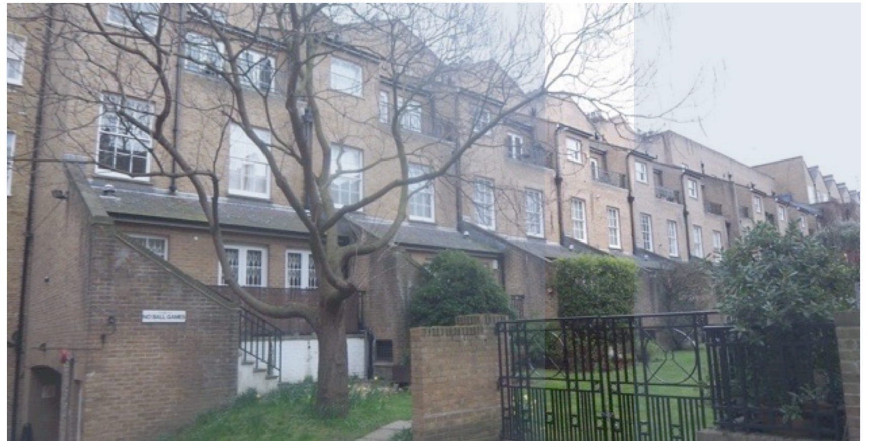
Rear Elevation, 67 Albany Street (highlighted), Rear Ground floor, late 20th C ground floor extensions, basement car park below.
