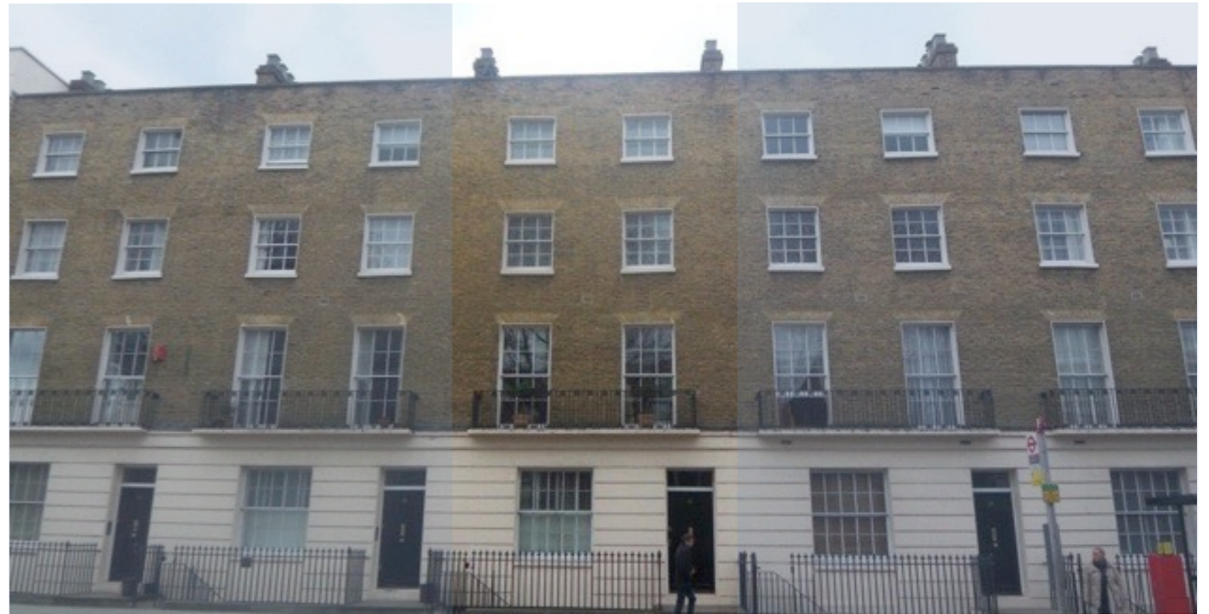
Front Elevation, 67 Albany Street (highlighted), 19th C terrace, restored 20th, Grade II listed.
