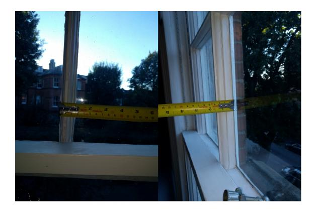
The new glazing to the windows will be slimline double glazed units, as such the new glazing bars to the new windows will match those as above in size and style.
