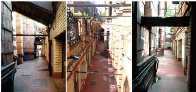
Existing Perimeter Lightwell, Russell Square
