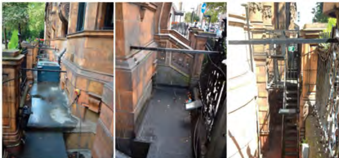
Existing Perimeter Lightwell, Guilford Street – showing area of infill
