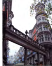
'Scillon Avenue' Market Entrance, Southampton Row
