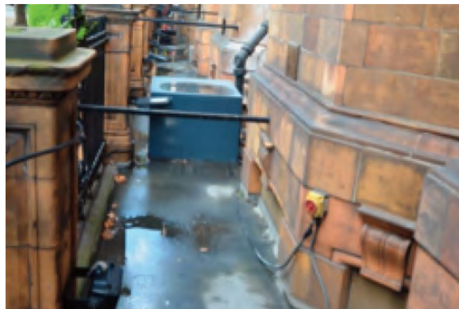
Figure 17: Infilled area in the Perimeter Lightwell on Guildford Street.
