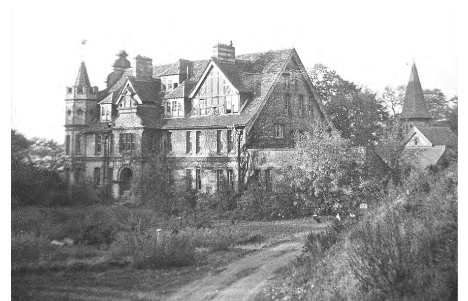
Figure 13: Photograph of Hadham Towers in Much Hadham, Hertfordshire. The residence was designed by Doll and where he ultimately retired to (Saunders, R., The Towers, Much Hadham, 18 December 2010, Flickr, www.flickr.com/ Accessed 16 March 2016).
