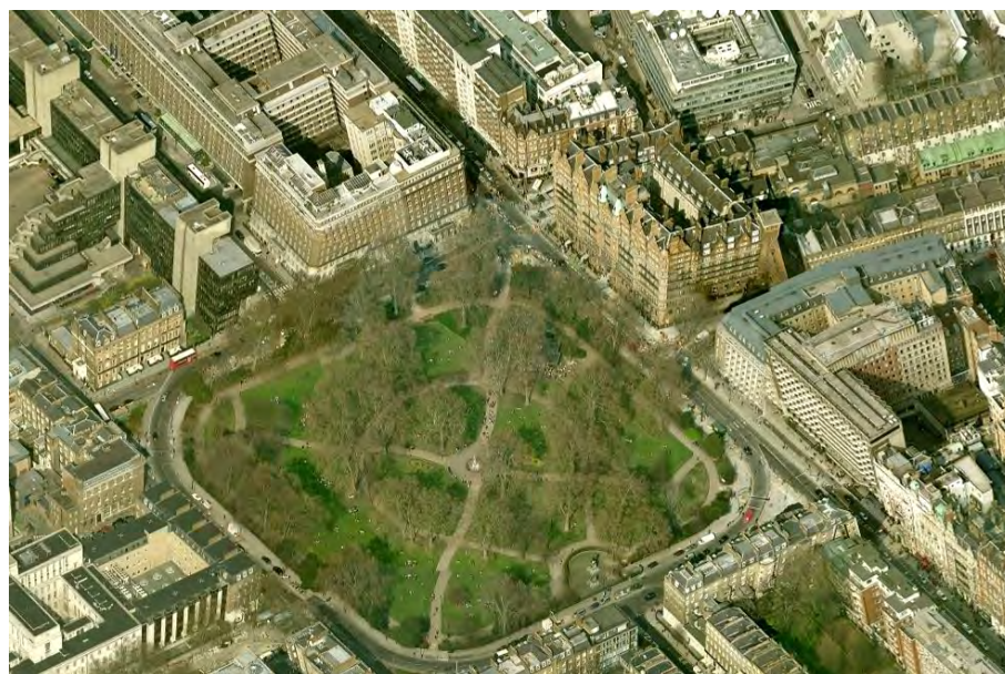
Figure 1: Aerial view of Russell Square where Hotel Russell is in a prominent location at the north east corner and facing onto Russell Square Gardens.
