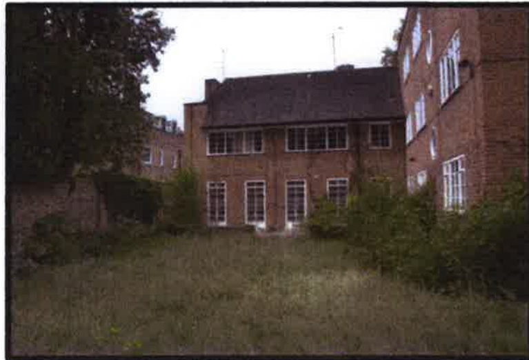
Picture showing the rear of the house.
