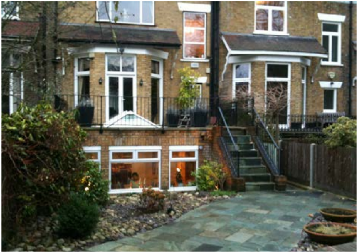
Image 1. Rear Elevation facing west
