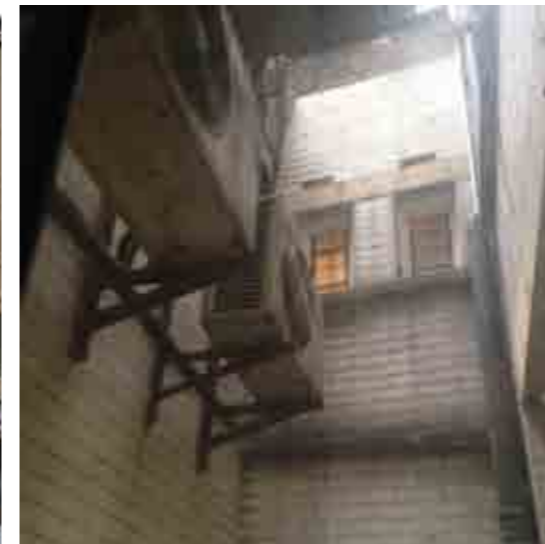
Existing South Courtyard - view from basement
