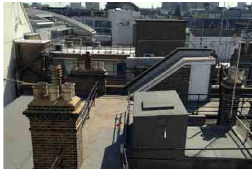
3_ 11.03.216 - View from the stair of the 5th floor looking the rear of the building
