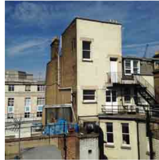
Existing South Courtyard - view from roof
