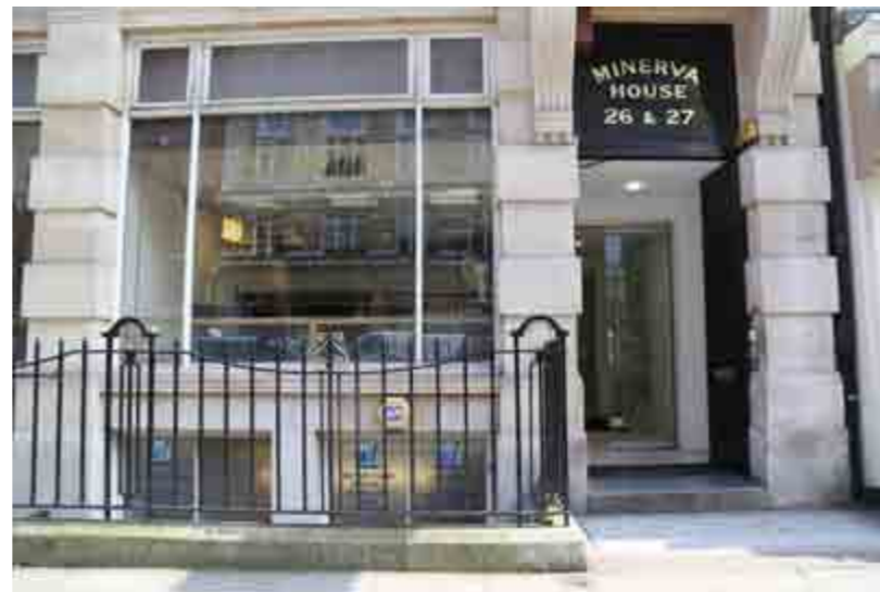
2_ 11.03.216 - Hatton Garden - existing entrance
