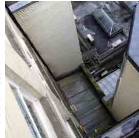
Existing North Lightwell - view from roof
