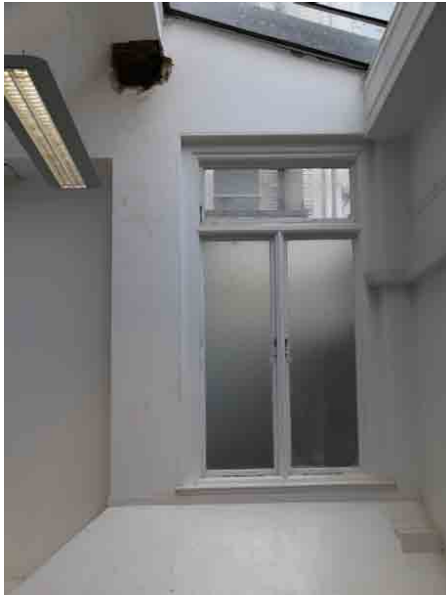
1_ 02.06.215 - View from ground floor to the lightwell
