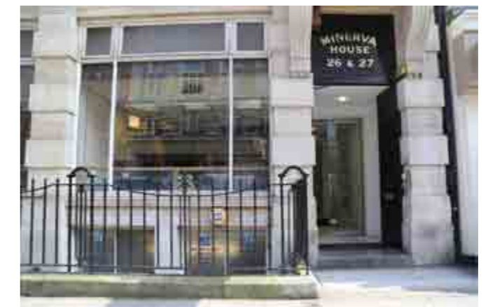
Hatton Garden - existing entrance
