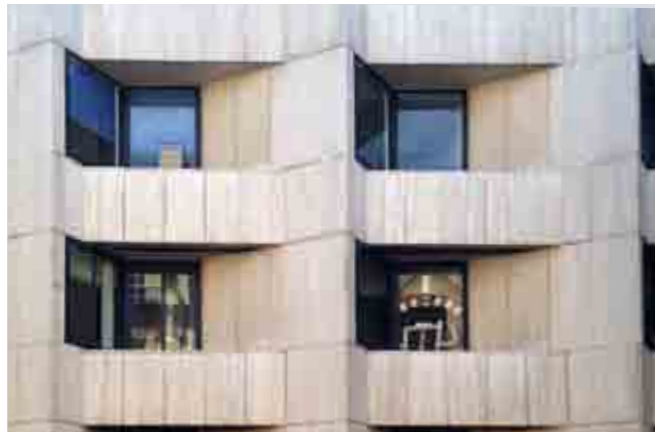
Jeygrove Court, 101 Hatton Garden - Travertine
