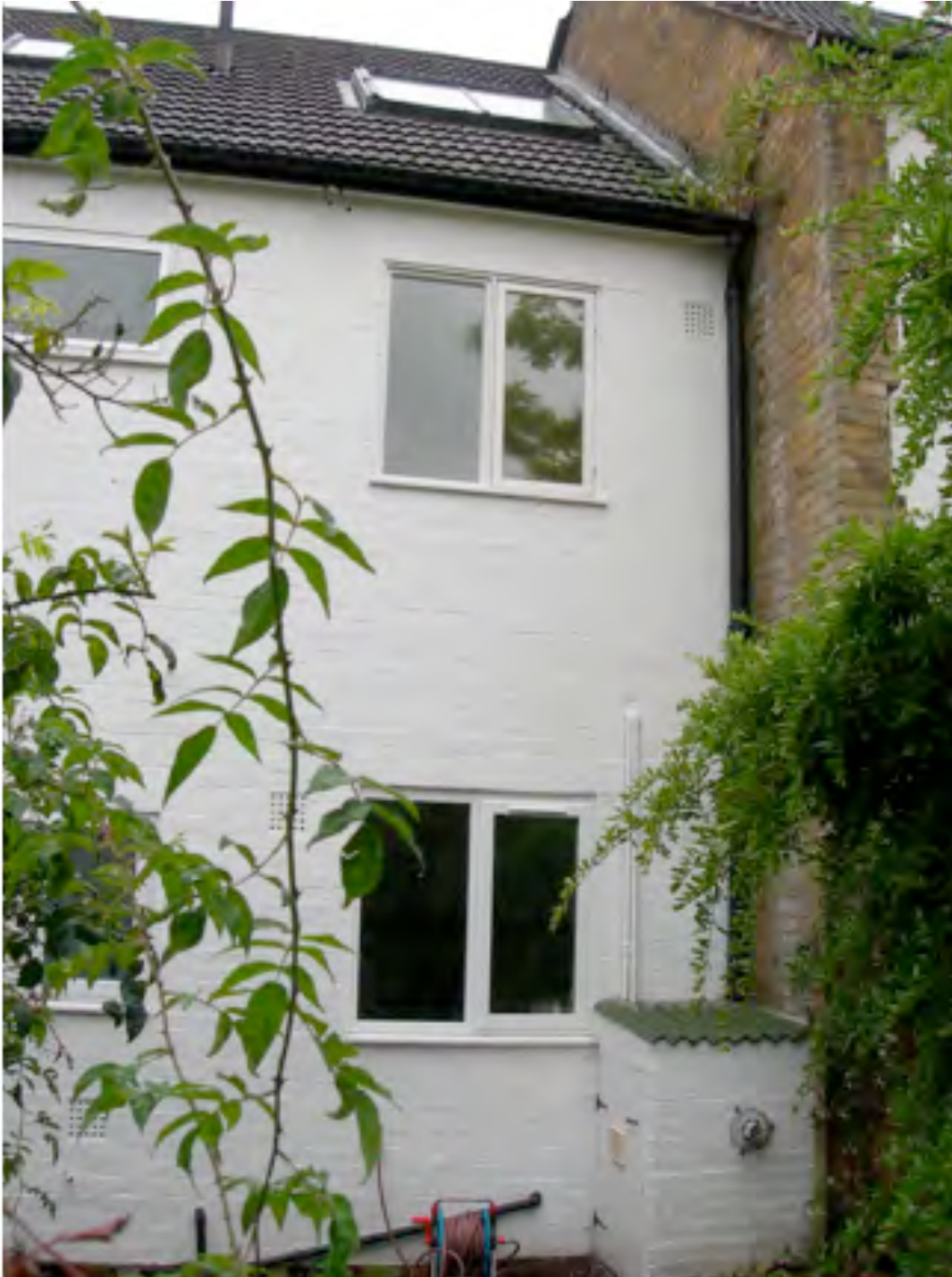
39 Rudall Crescent- Rear Elevation
