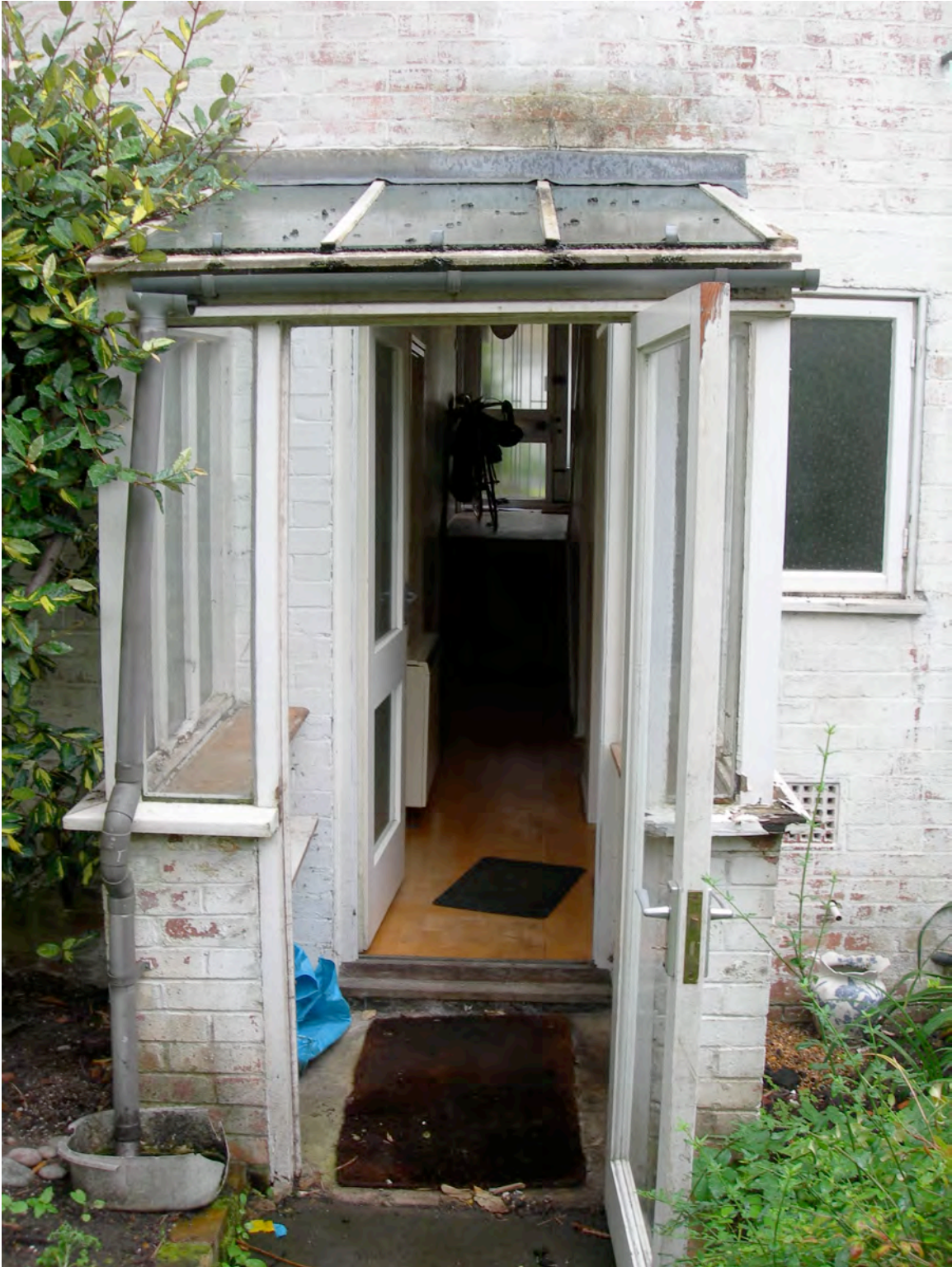
37 Rudall Crescent- Rear Elevation
