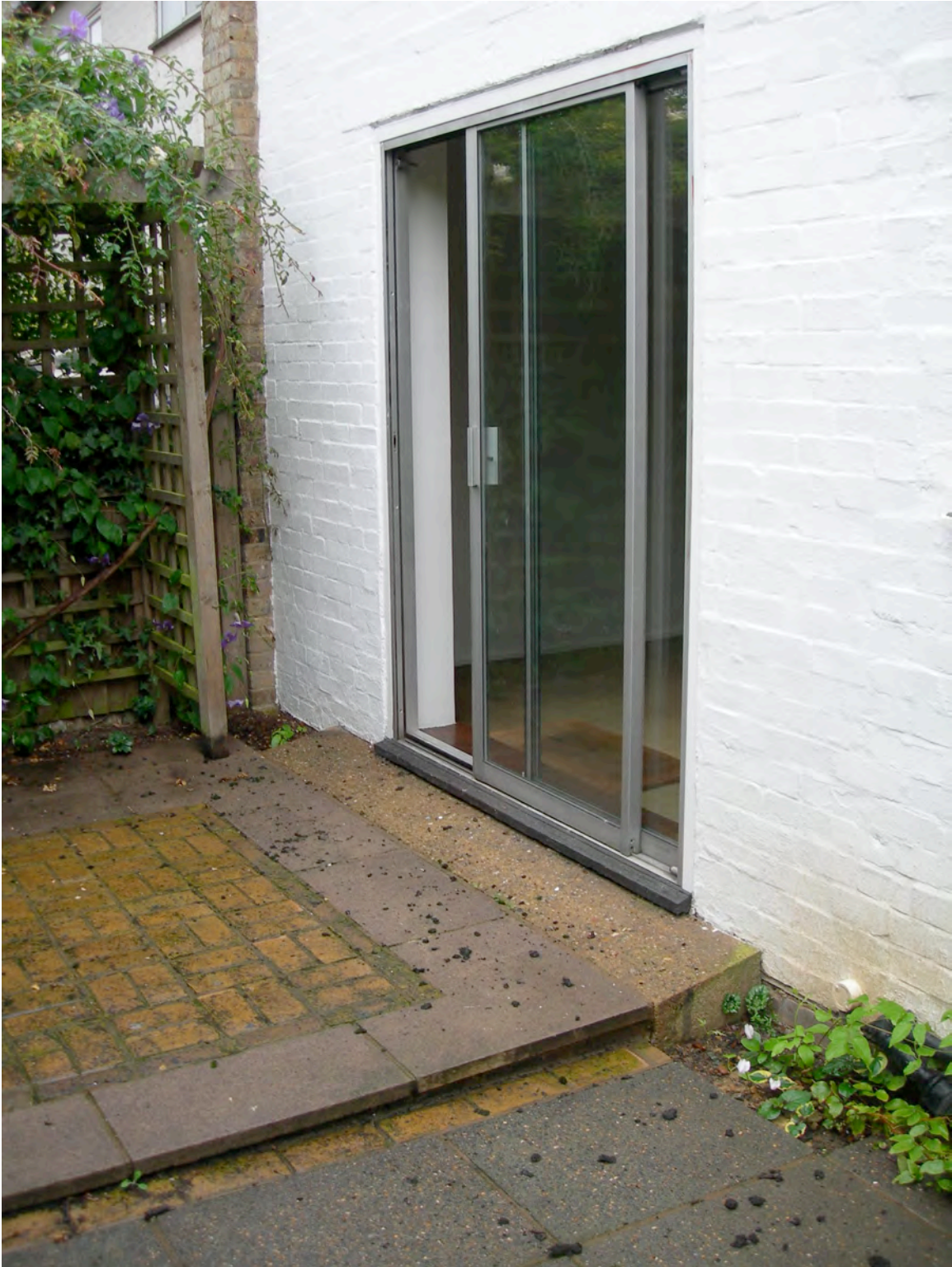
39 Rudall Crescent- Rear Elevation
