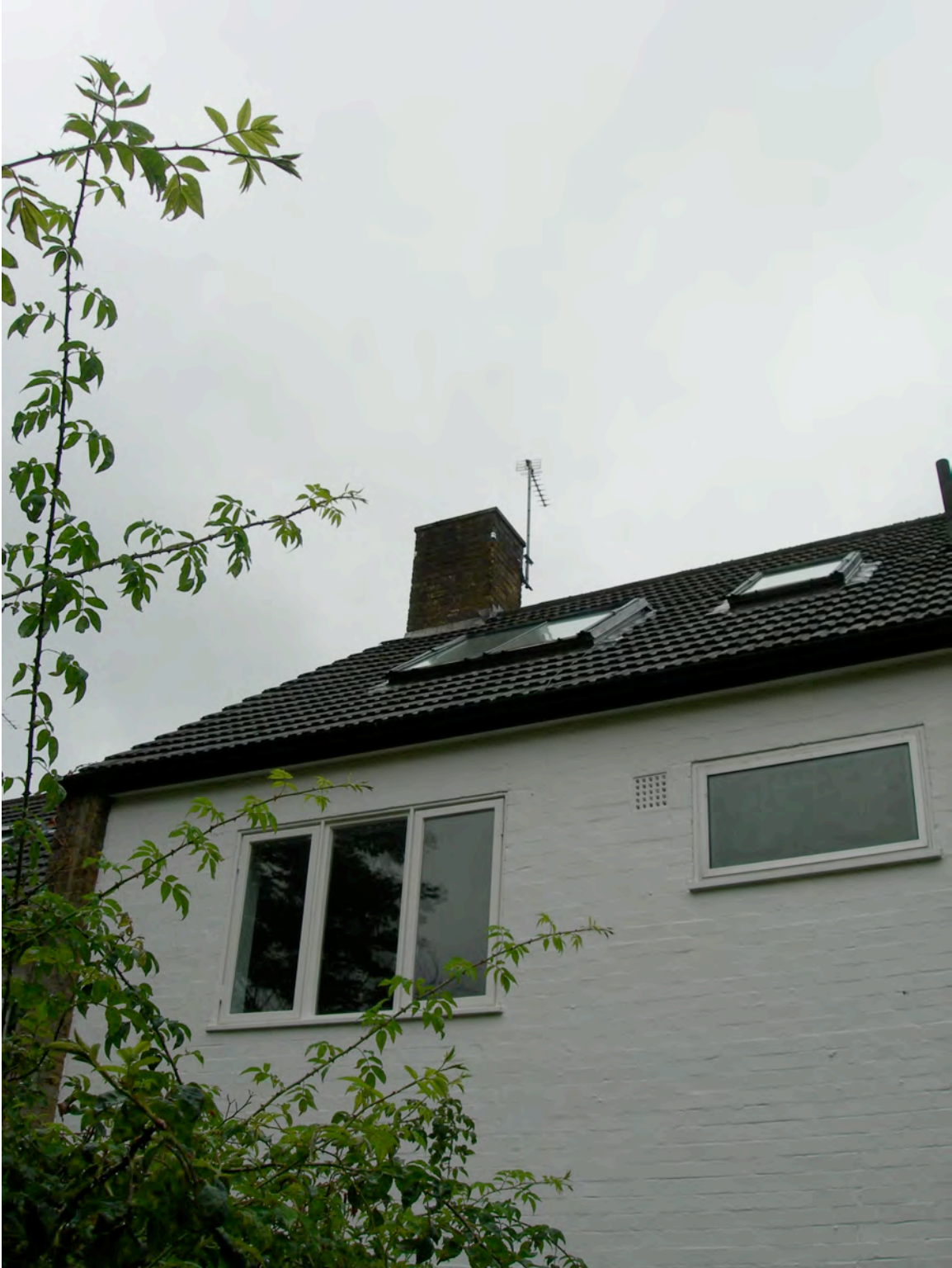
37 Rudall Crescent- Rear Elevation
