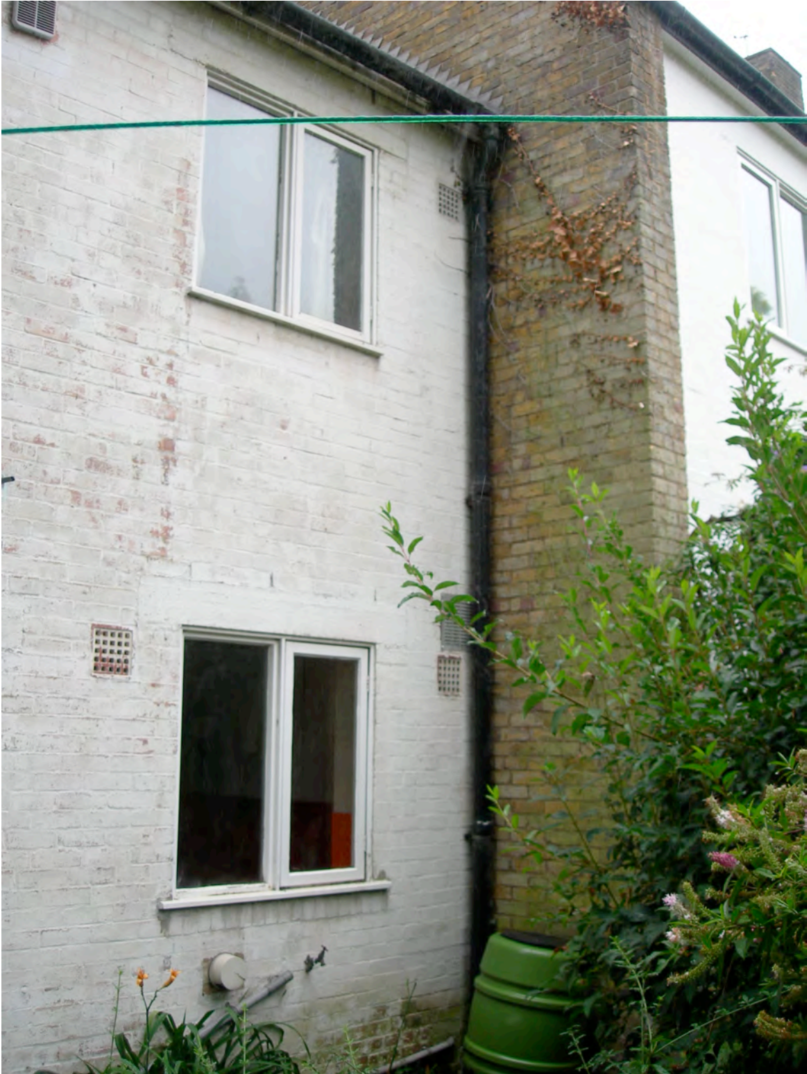
37 Rudall Crescent- Rear Elevation
