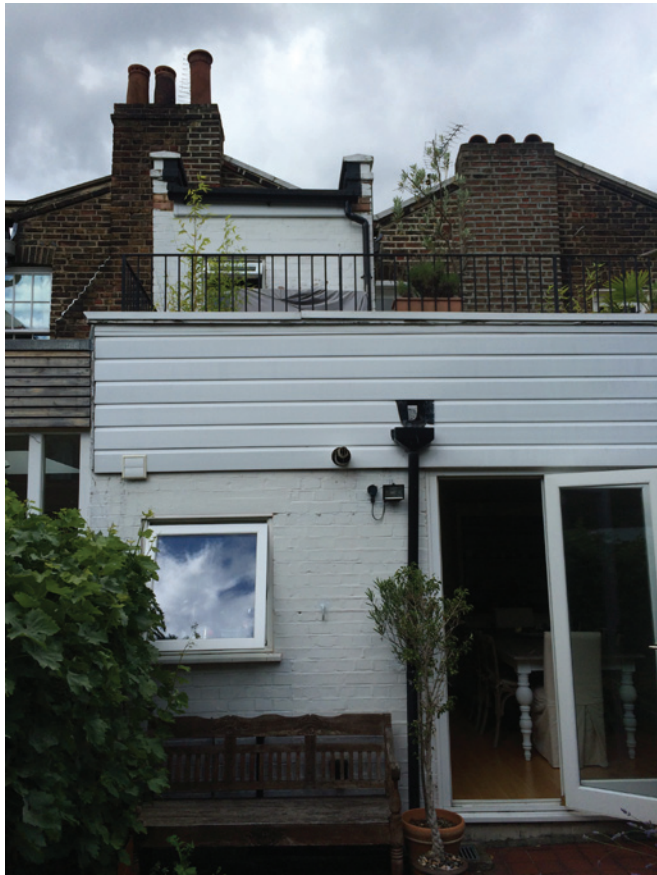
View from garden looking up at existing first floor terrace and bathroom
