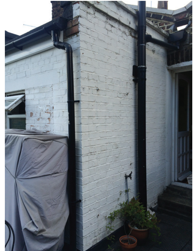
View of exterior of existing first floor bathroom.
