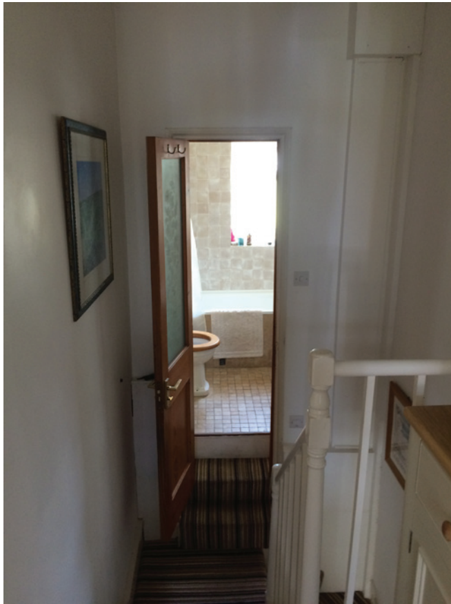
Interior view looking towards bathroom entrance with door opening immediately onto stairs.
